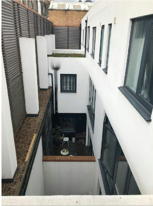
View looking North West across both courtyards of 5 & 6 Whittlebury Mews West, showing tall retaining (party wall) between the Whittlebury West and Gloucester Ave properties.
