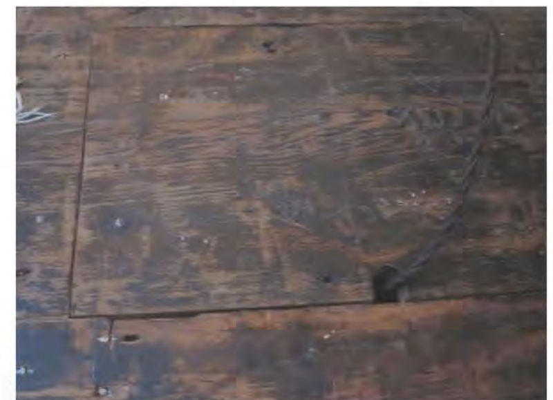
FLOOR BOX IN FLOOR BOARDS
