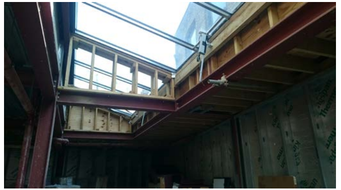
Ground floor roof lights
