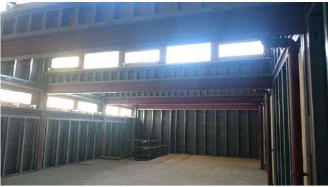
First floor level showing roof lights
