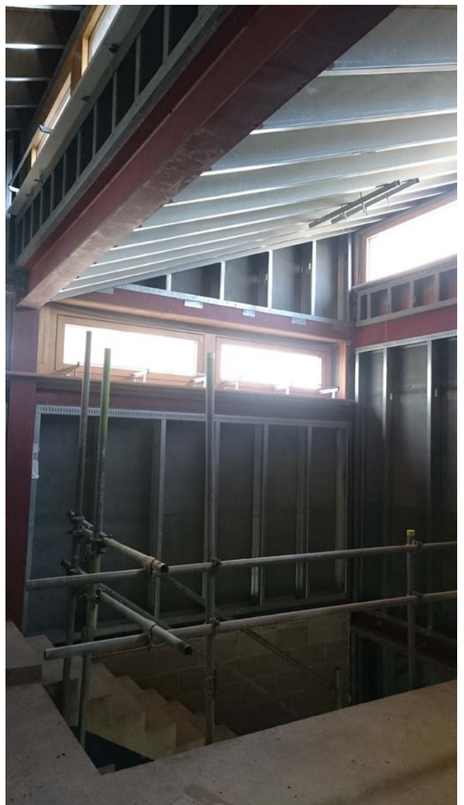
Stairwell at first floor level
