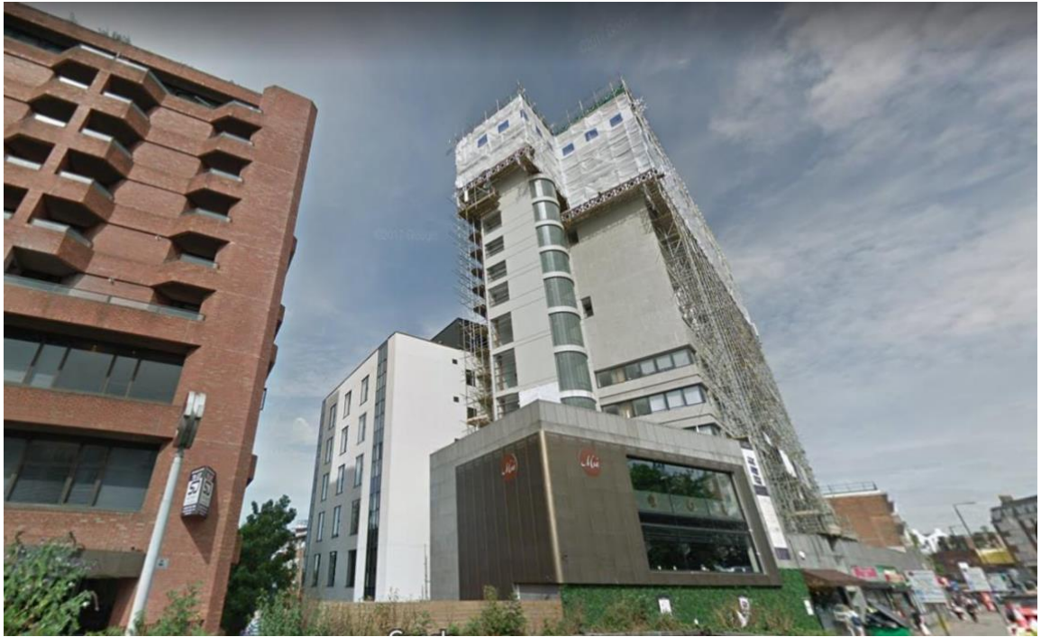
Photograph 2 – 135 Finchley Road –Perforated Aluminium cladding installed
