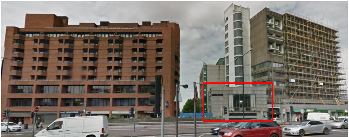
Photograph 1 site photograph of 135 Finchley Road outlined in red - Prior to the installation of the perforated aluminium cladding.
