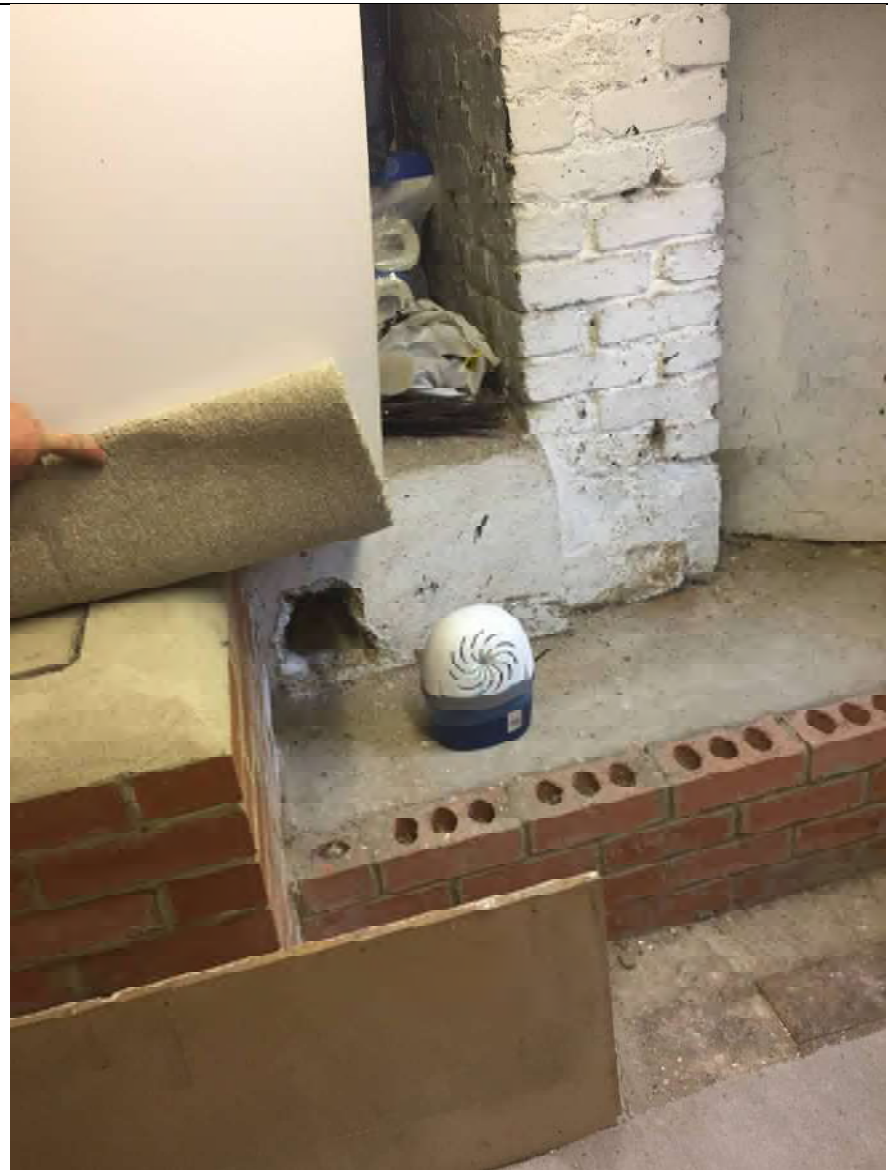
Plate 4: Drain cover within existing basement/cellar.
