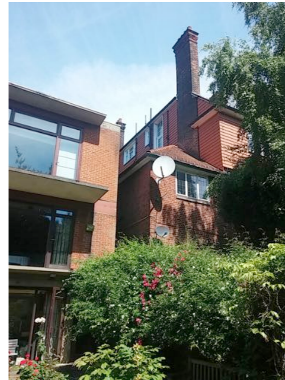
View from garden at Nos.56 & 58a Redington Road
