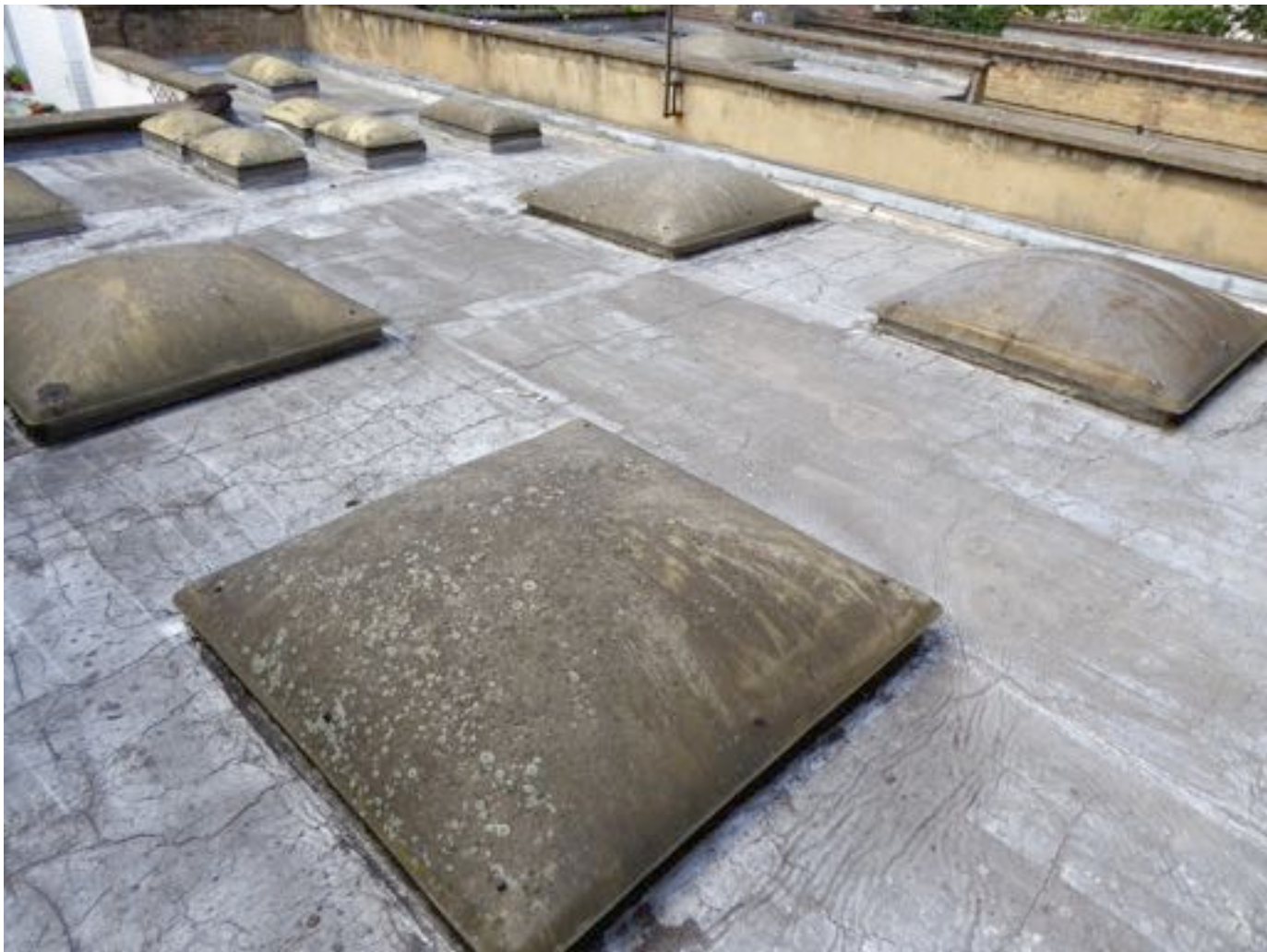
Photograph of the life-expired polycarbonate domed roof lights over 4 Lamp Office Court.
