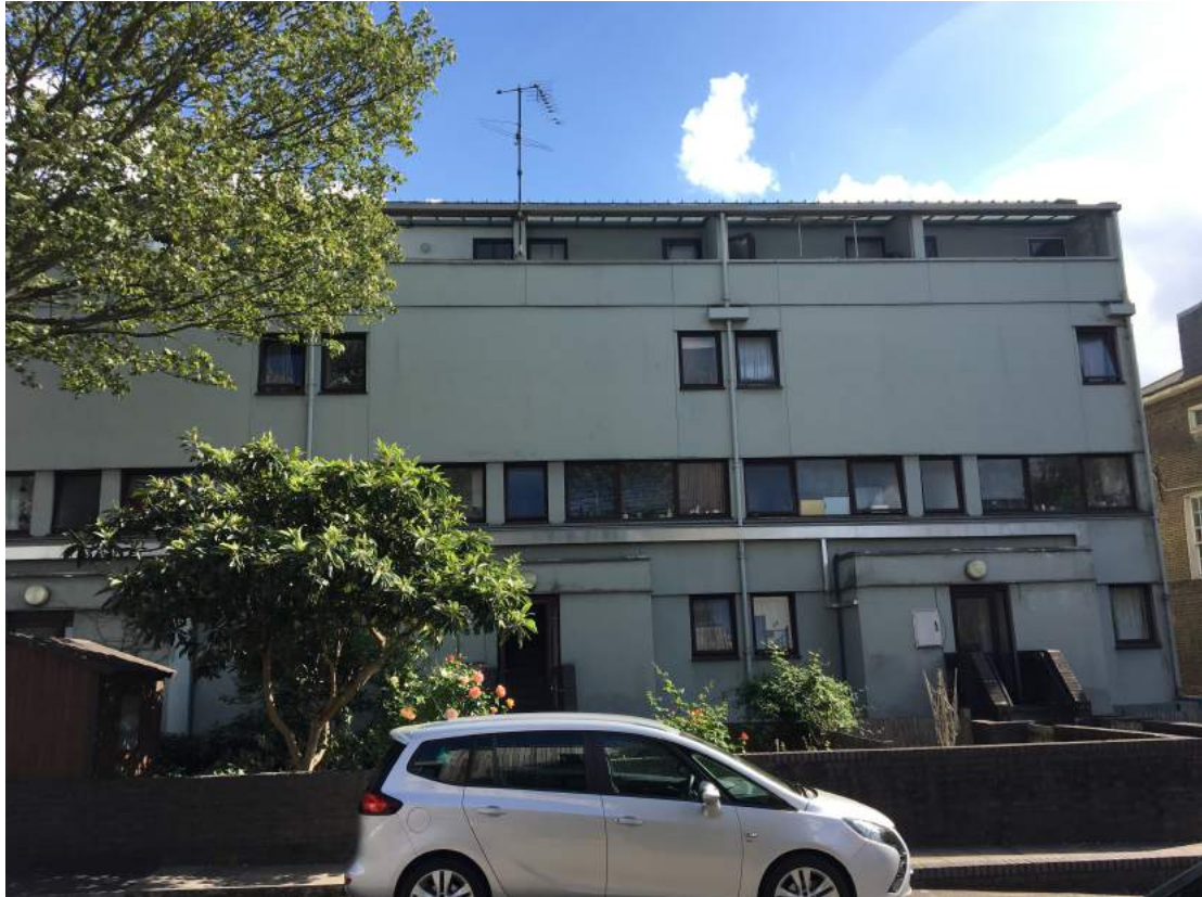
Existing rear elevation 217-225 Camden Road
