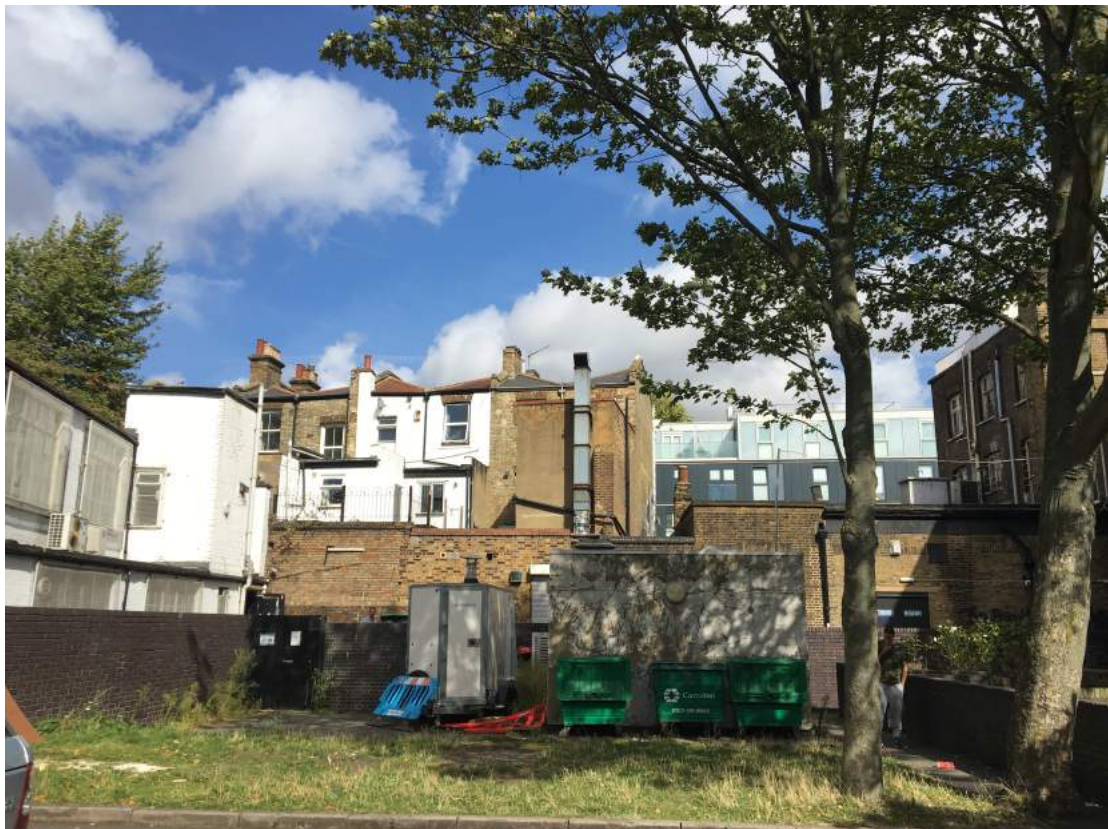
Existing surrounds and bin storage units
