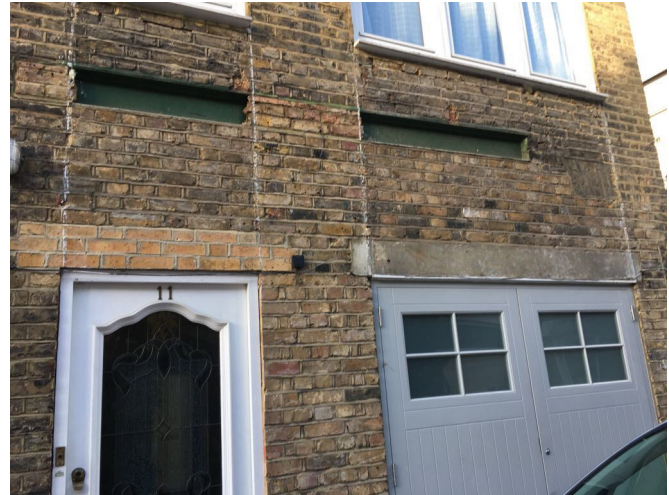
Differing brickwork, steelwork & concrete
