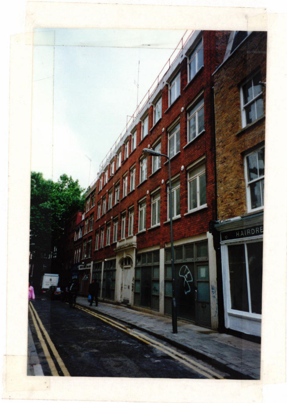
Laystall Street Elevation (Viewed from southern end of Laystall Street)
