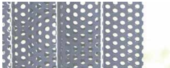
03 Perforated grey metal cladding
