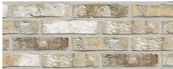
01 Brick to approximate the London stock brick used to rear of neighbouring mansion blocks
