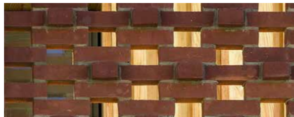
03 'Hit and miss' brickwork
