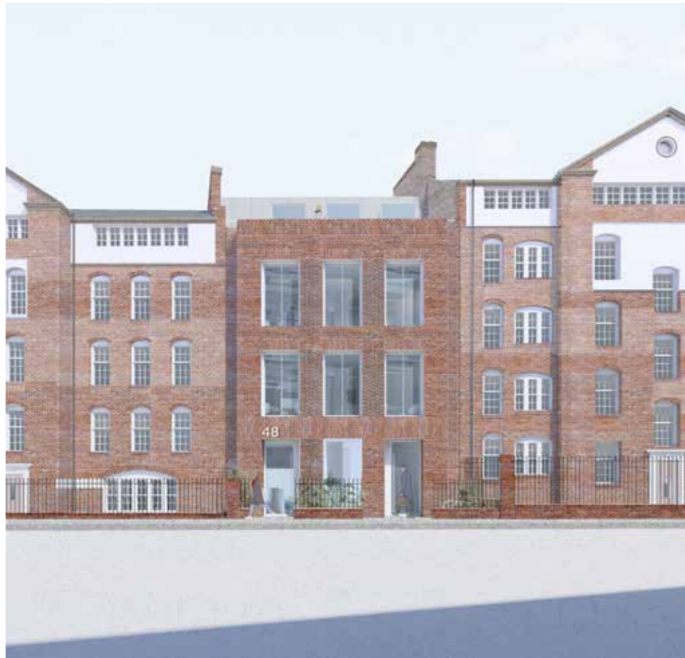
01 Red brick with symmetrical ground floor piers
