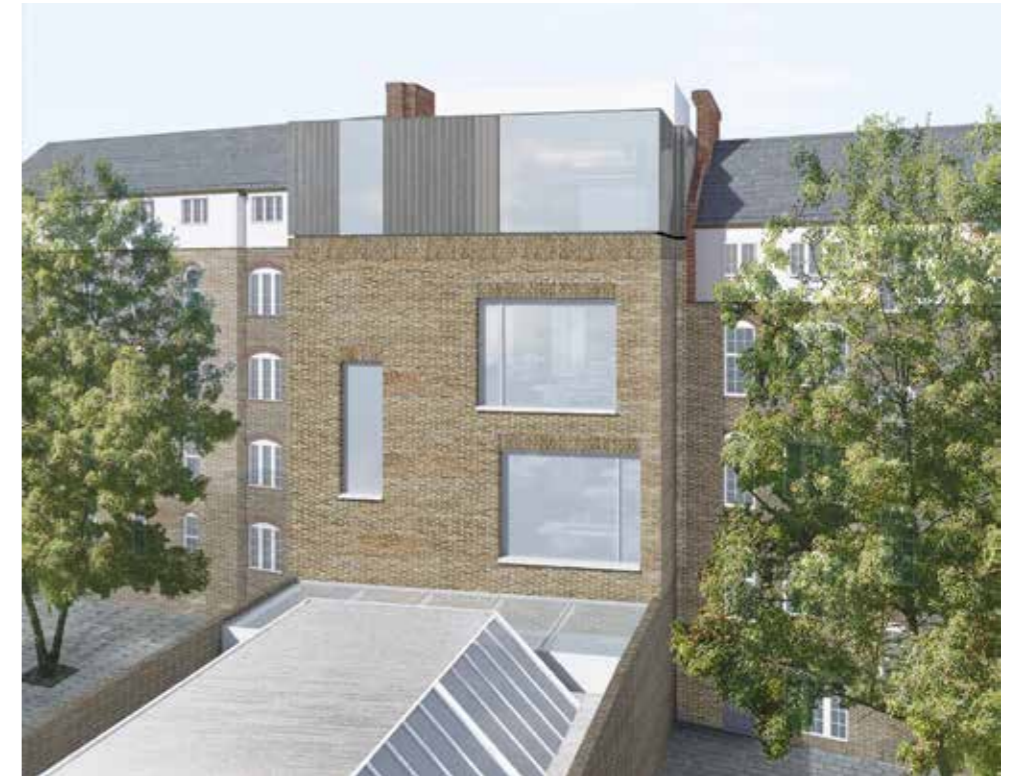
06 Single stair landing window and aligned upper stair window, with larger, misaligned recessed openings to the office floors. Opening casements to first and second floor, and perforated dark metal cladding to third provide natural venting to the offices.
