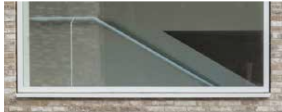
02 White anodised aluminium frames
