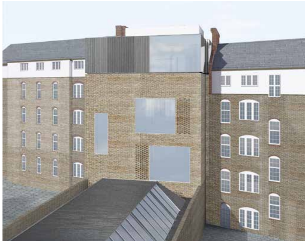
04 Single stair landing window and aligned upper stair window, with larger misaligned openings to the office floors. 'Hit and miss' brickwork to first and second floor, and perforated dark metal cladding to third provide natural venting to the offices.
