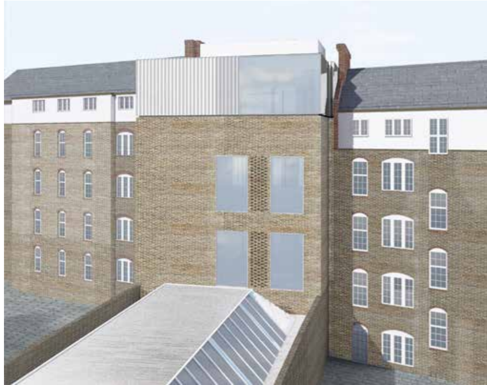
01 Blank wall relative to stair core, with vertically aligned window openings to office floors. 'Hit and miss' brickwork to first and second floor, and perforated metal cladding to third provide natural venting to the offices.
