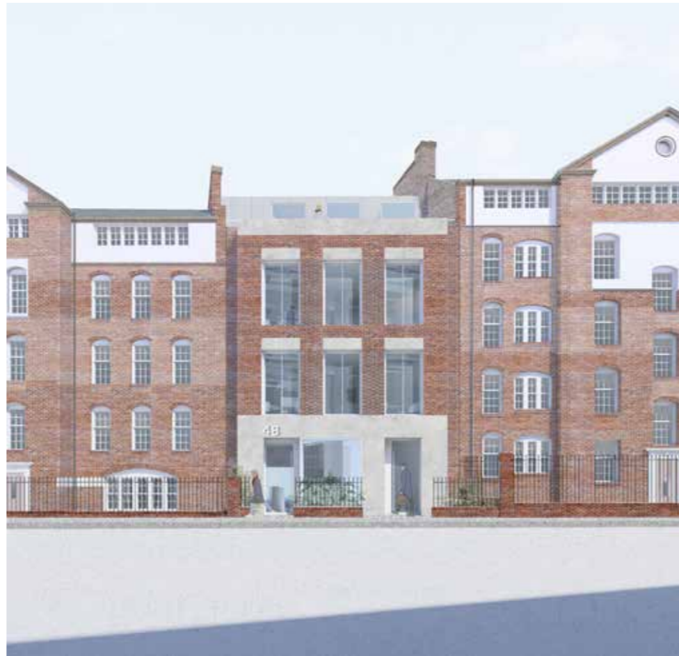
05 Red brick with an expressed concrete base and head details
