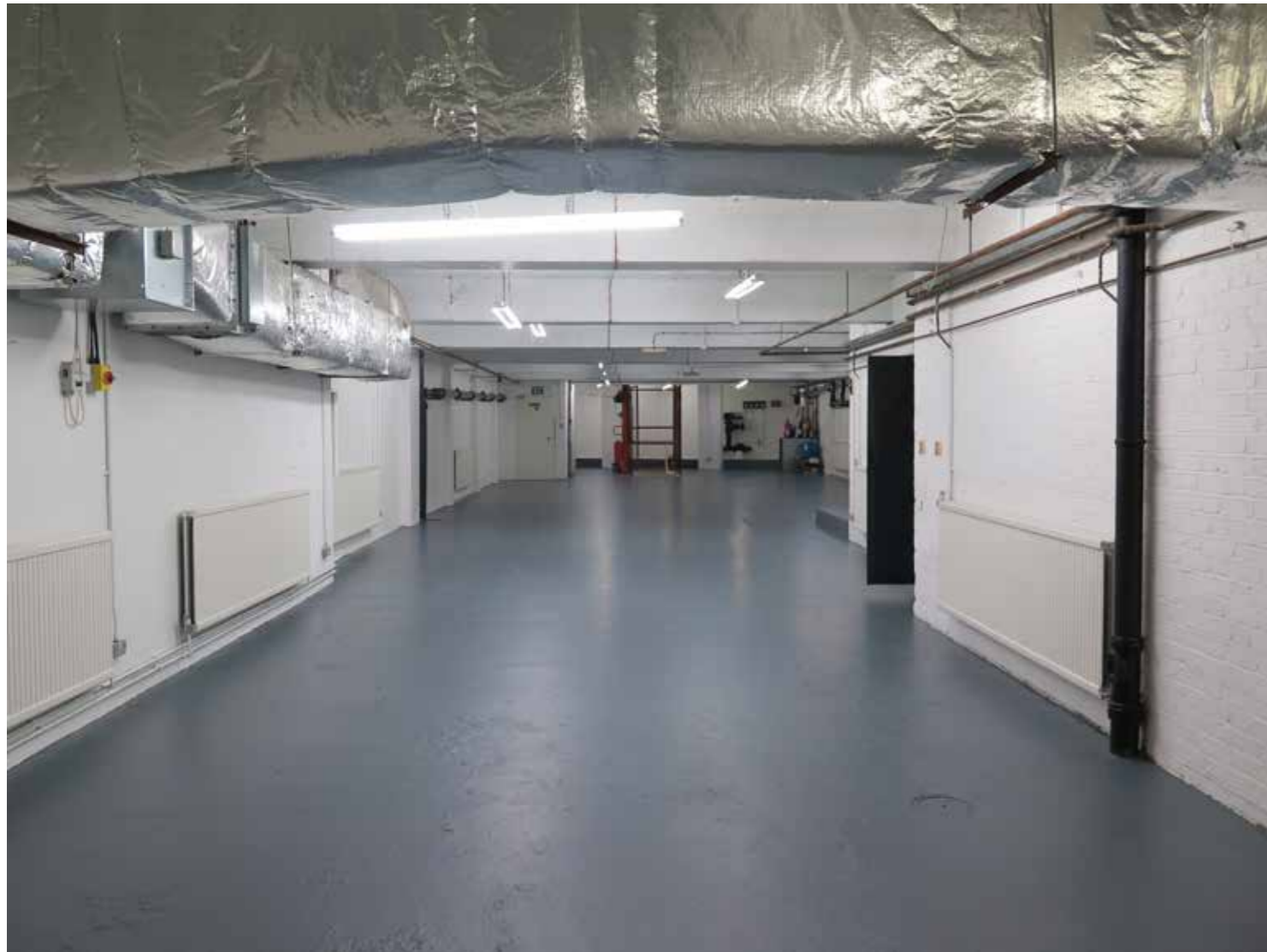
Basement level looking east
