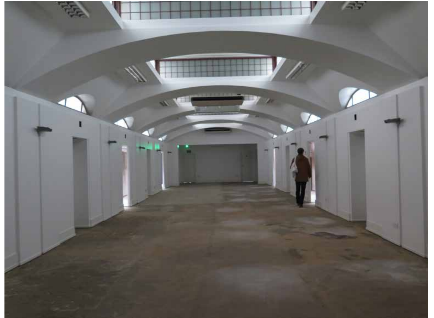
Open plan space that forms the majority of the existing ground floor area, with post-modern fit-out and service voids to the perimeter
