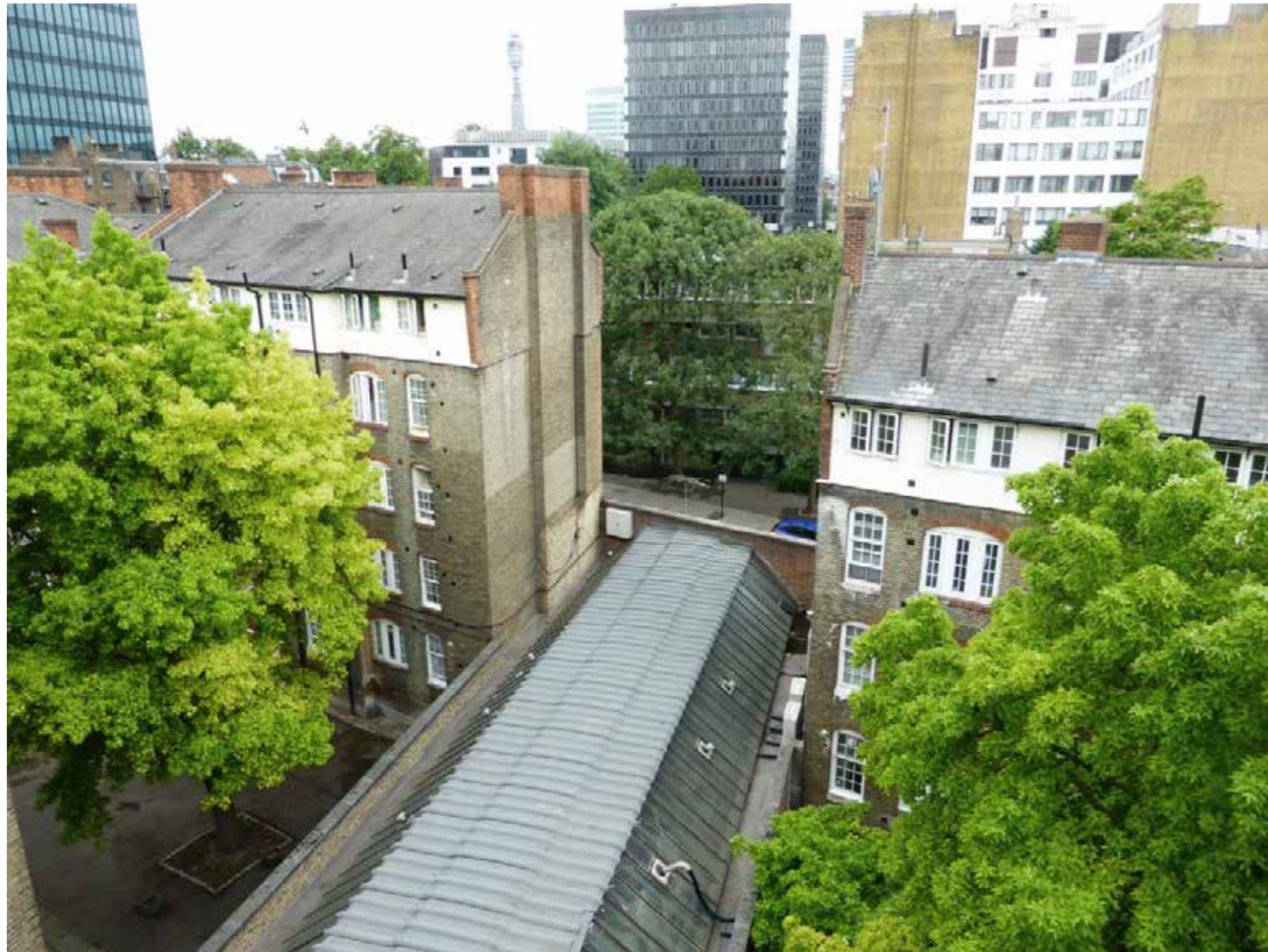
Existing roof looking west
