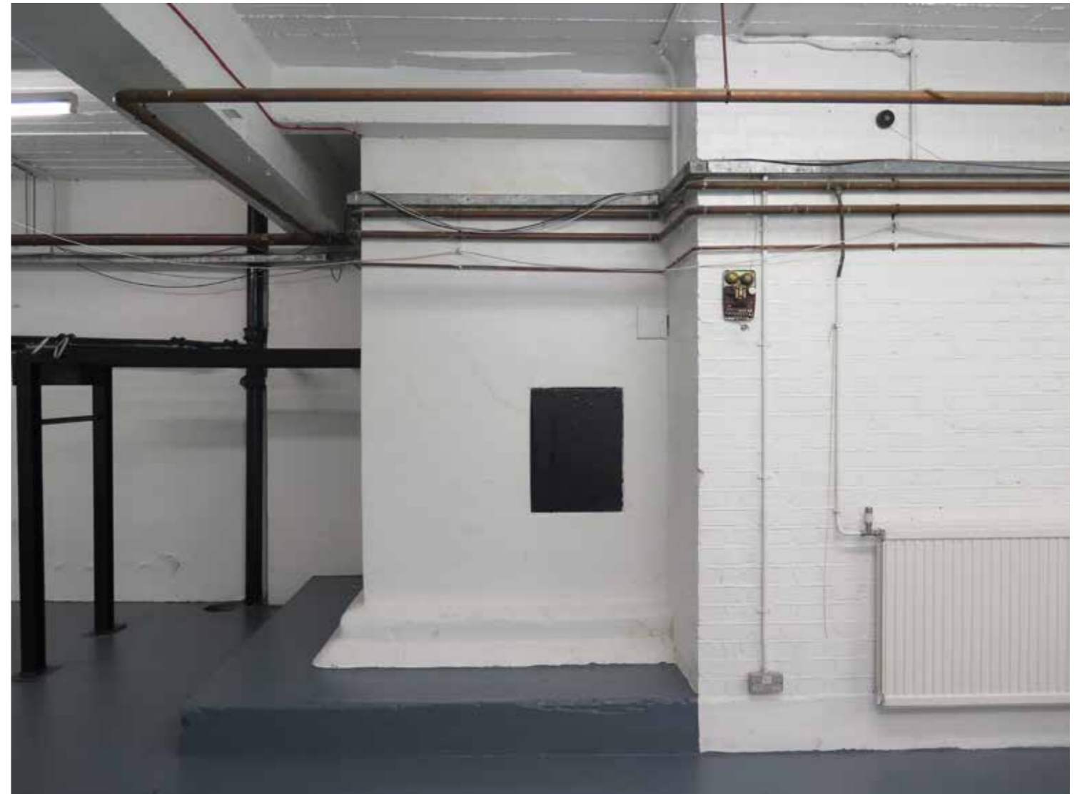
Services currently characterise the ceilings and walls at basement level
