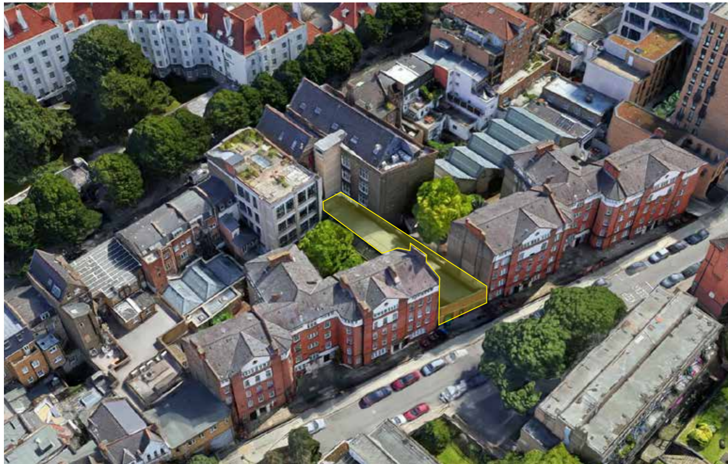
Overview of the site looking south east
