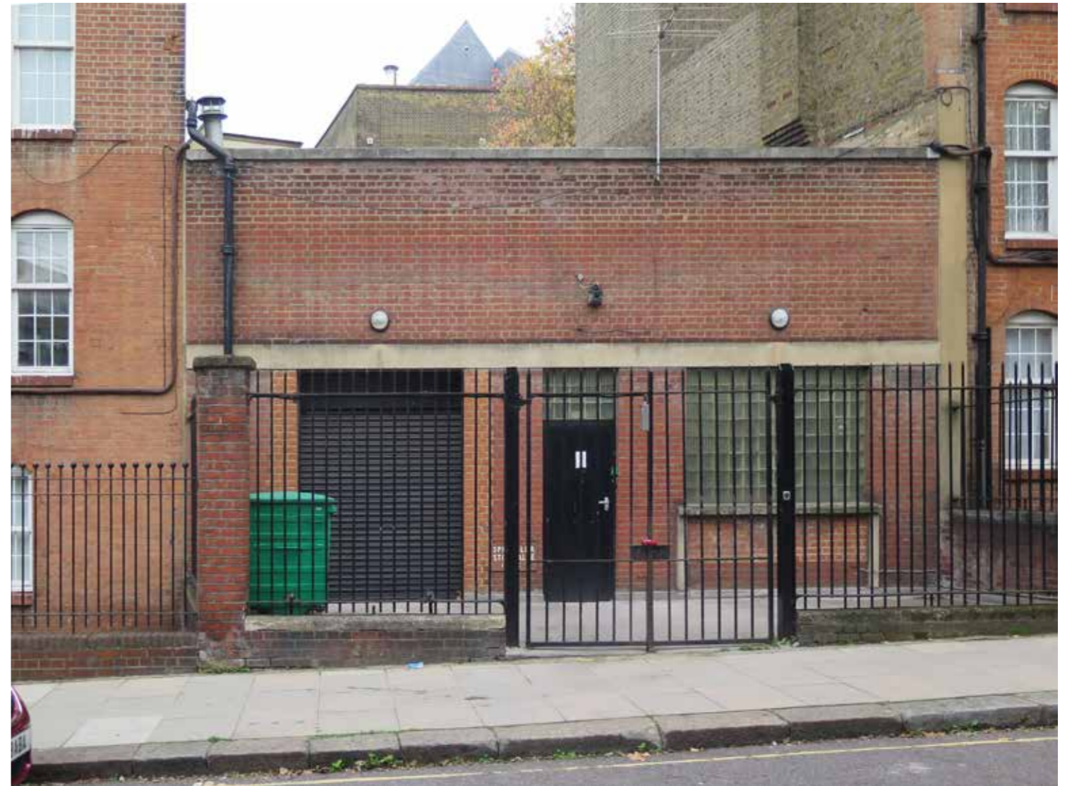
Churchway looking east at the site
