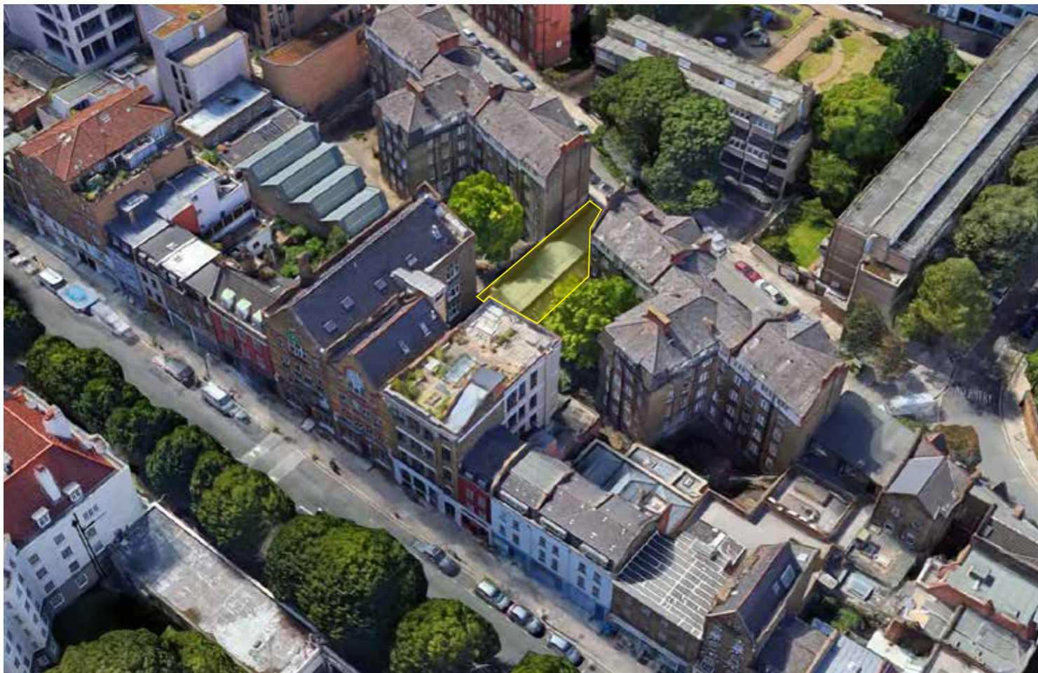
Overview of the site looking south west
