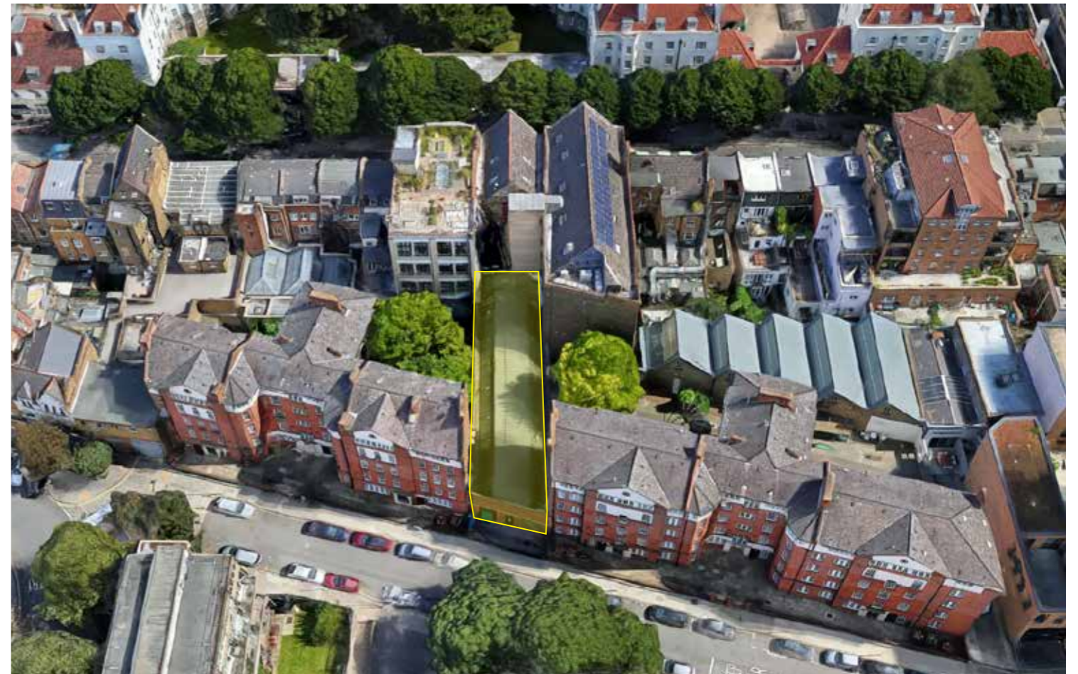
Overview of the site looking east
