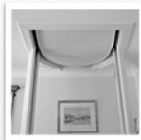
View of downstairs looking up at underside of the lift.
