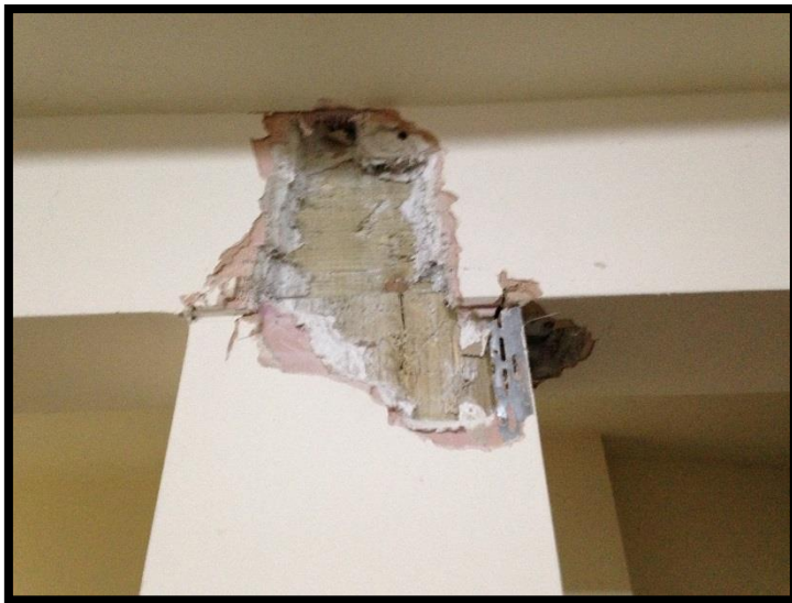
Exposure of timber members forming the support feature
