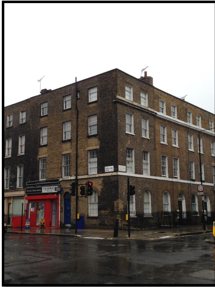
General view of front and right-hand elevations
