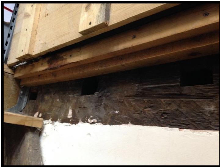
Original beam above support feature – note horizontal mortice
