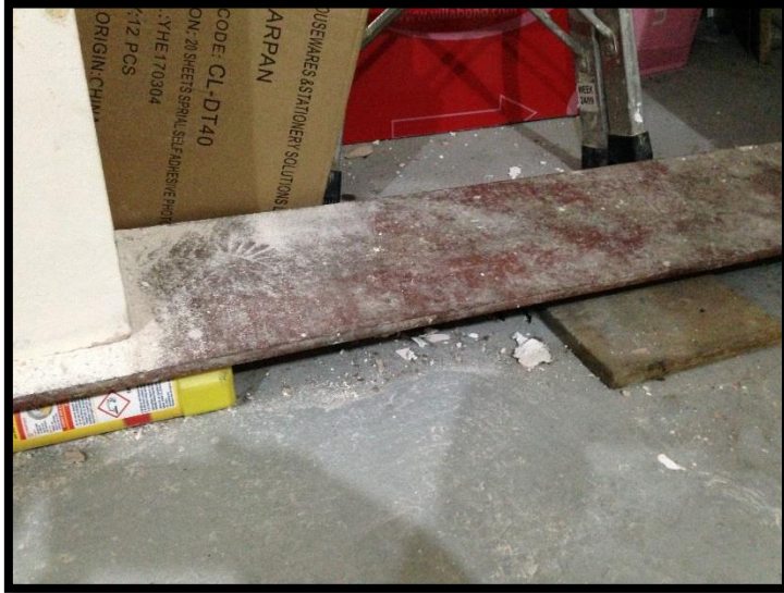
Steel beam embedded in basement floor
