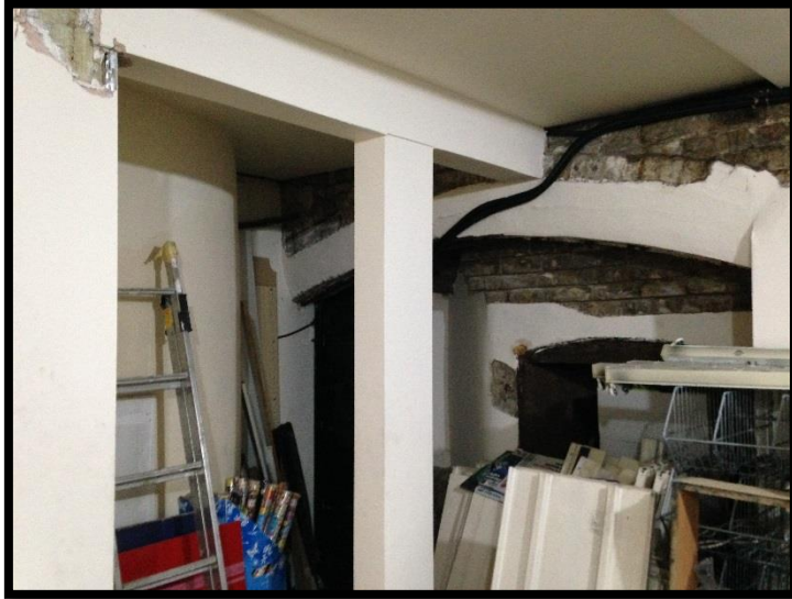
Support feature close to front wall and arch
