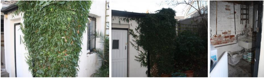
EXISTING REAR EXTENSION
