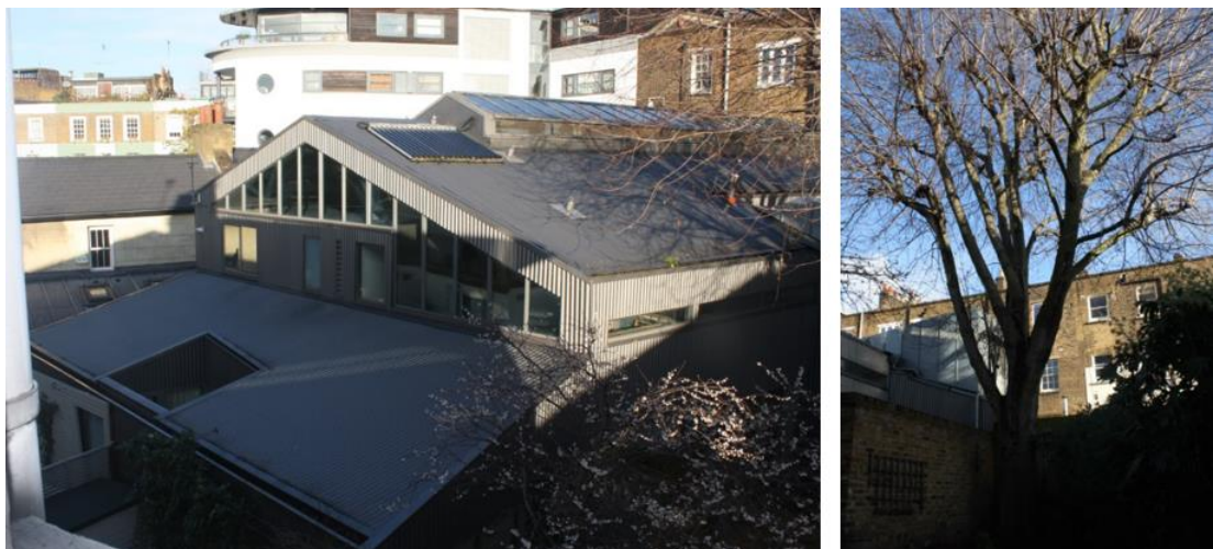
LIVE-WORK BUILDING (LEFT) AND SILVER MAPLE (RIGHT)
