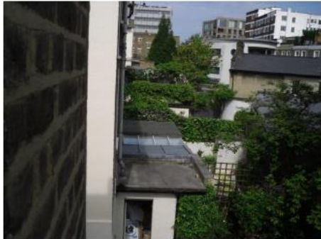
Single storey extensions at basement level
