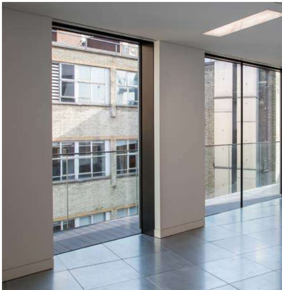
External Glazing Silicone jointed large format clear glazing system to office levels
