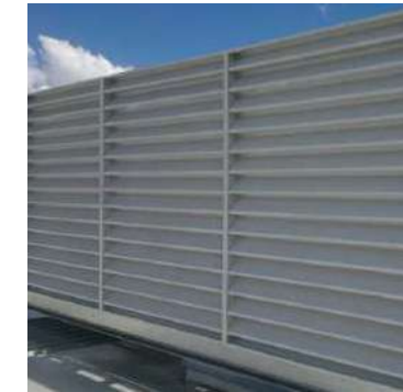
Louvred Plant Screen PPC light coloured metal acoustic louvred plant screen to roof plant.
