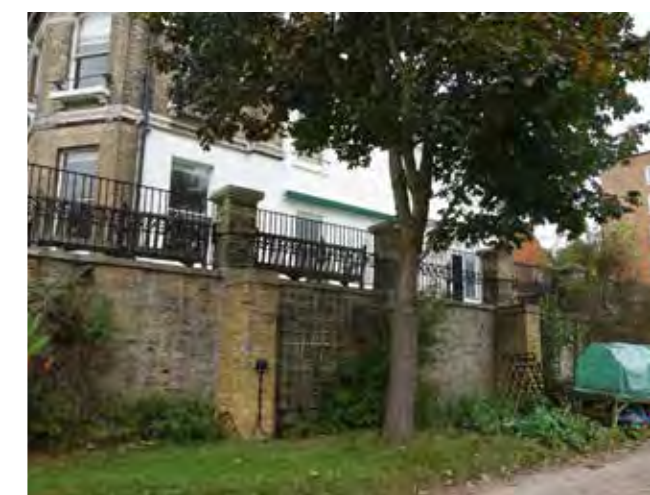
View of Existing Masonry Retaining Wall, East Elevation
