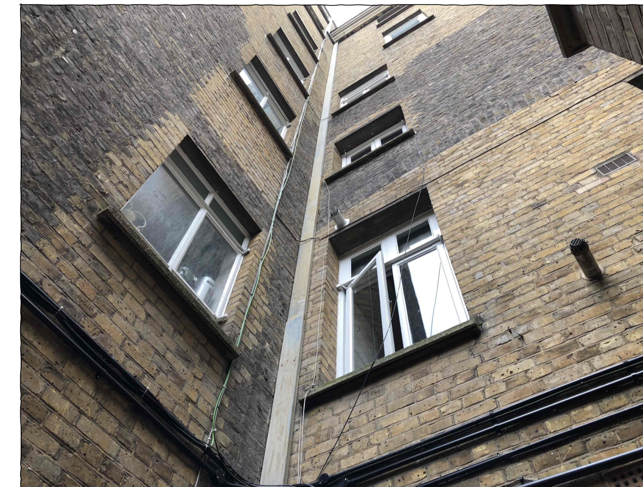
Photograph taken up from Basement Level Lightwell
