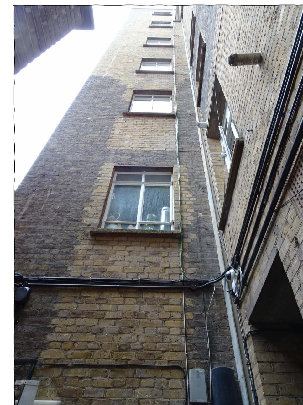
Photograph taken up from Basement Level Lightwell
