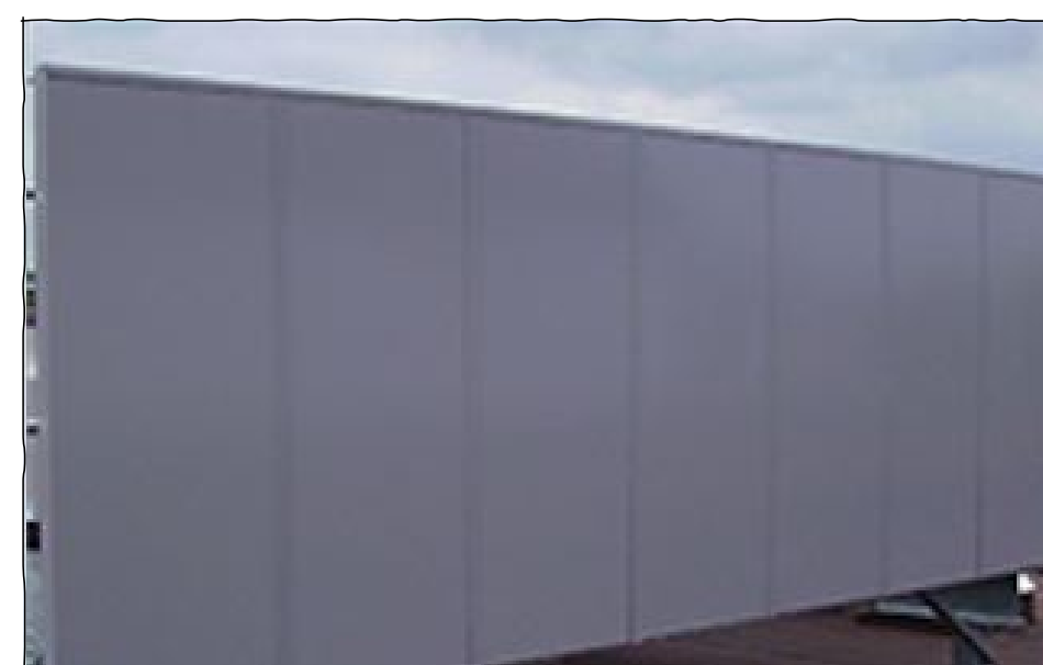
Proposed polyester powder coat finished Acoustic Screen Panel Type Finished in RAL 7040 'Gun Metal Grey'
