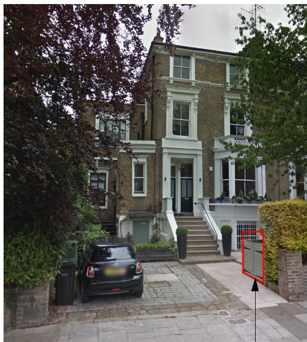
No. 11 bins located in open storage shelter
