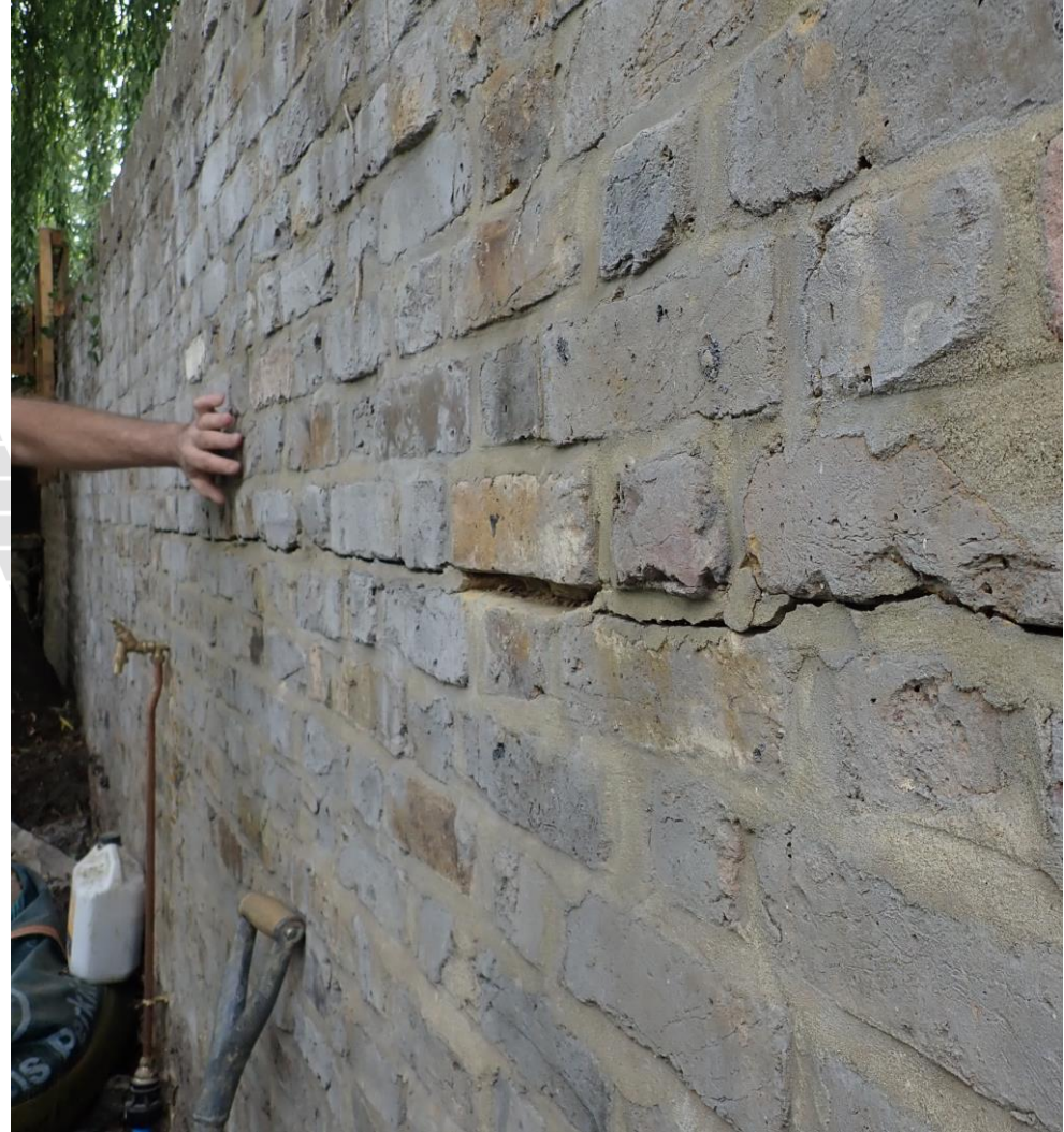
Left: vertical crack in west boundary wall at point where foundations change -position of future movement joint (left of this line proposed for careful deconstruction and rebuilding)
