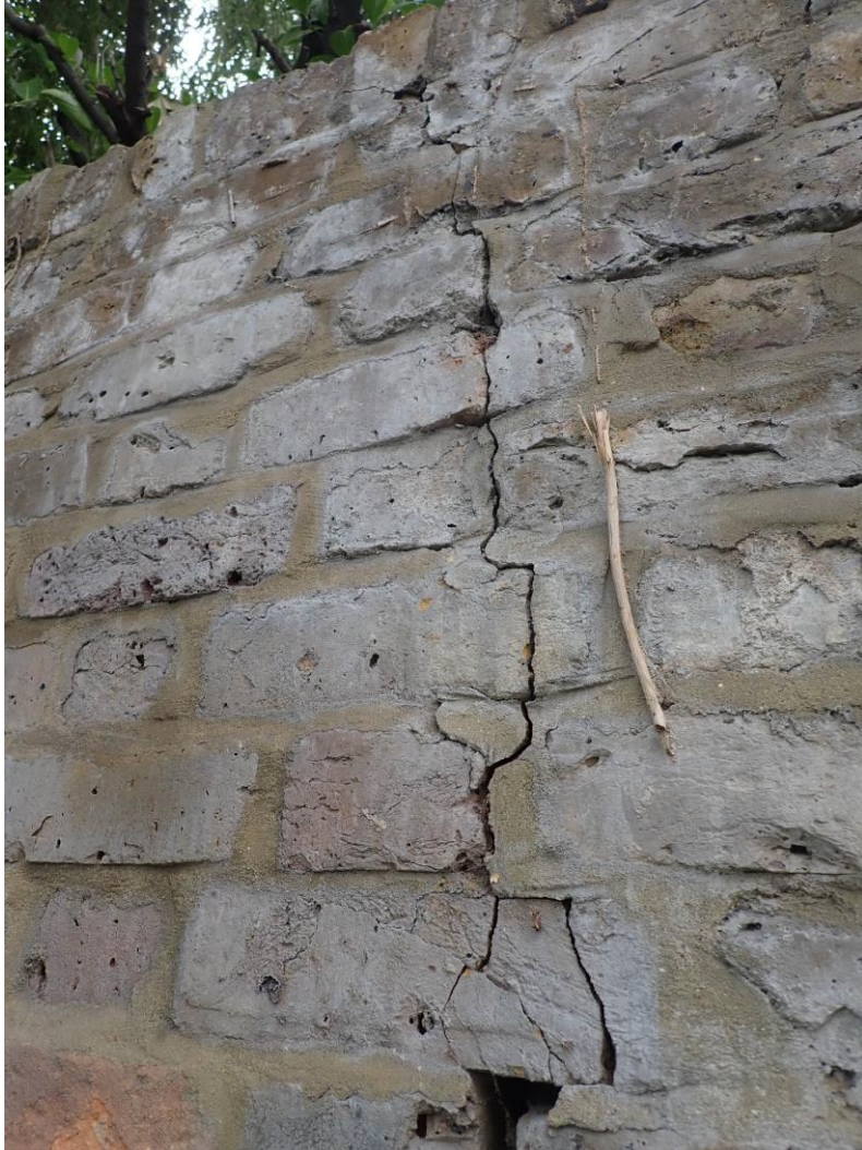
Left: vertical crack in west boundary wall at point where foundations change -position of future movement joint (left of this line proposed for careful deconstruction and rebuilding)
