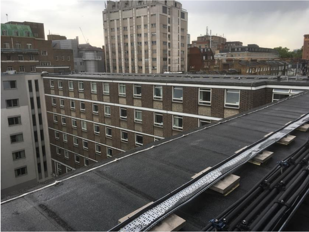
Photo of existing roof
