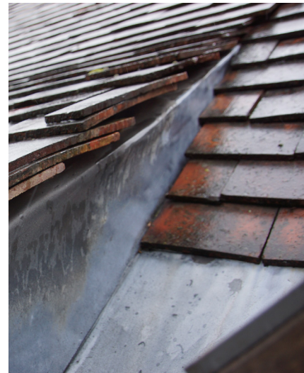
The tiles were originally terracotta colour but have weathered and become dark in colour.
