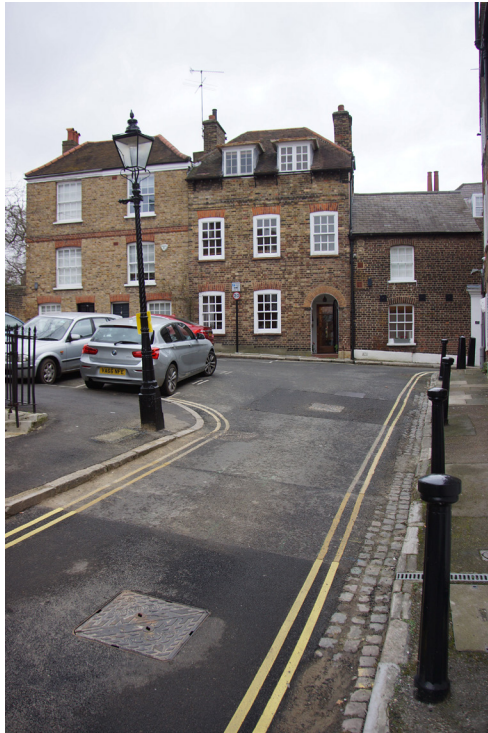
Front facade on The Mount Square.
