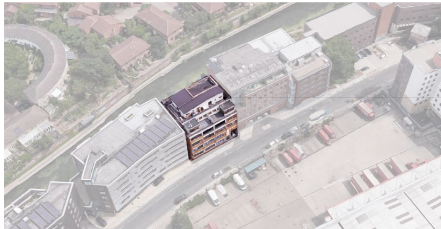
EXISTING BUILDING 18-20 ST PANCRAS WAY
