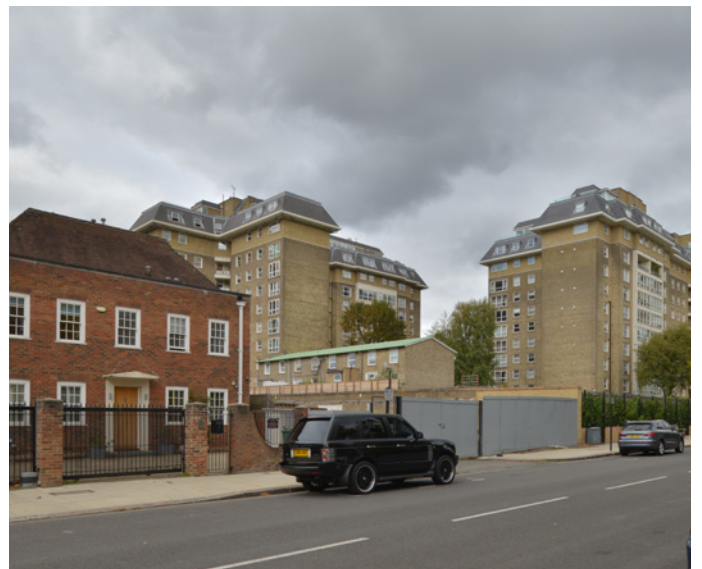
6.Site with Boydell Court in the background
