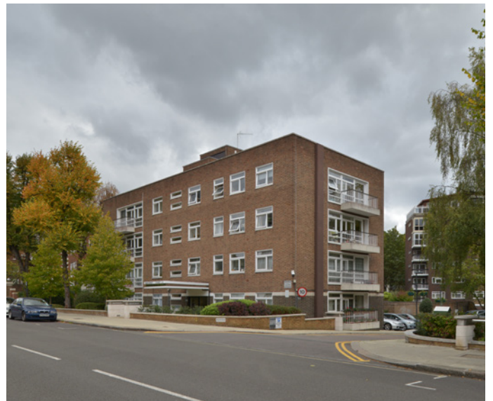
4.Mancroft Court opposite site
