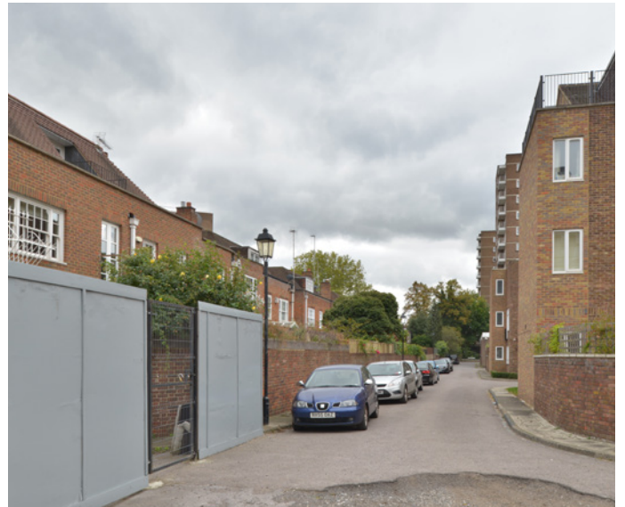
4. Rear of the site looking towards north
