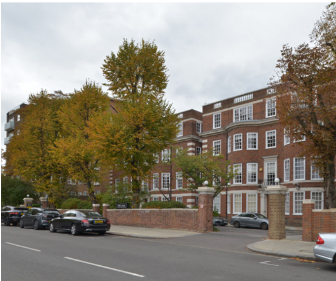
3.Park Lodge opposite site
