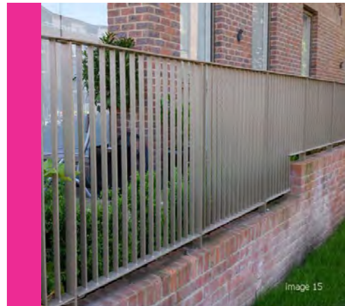
Brick wall & flat top railing
