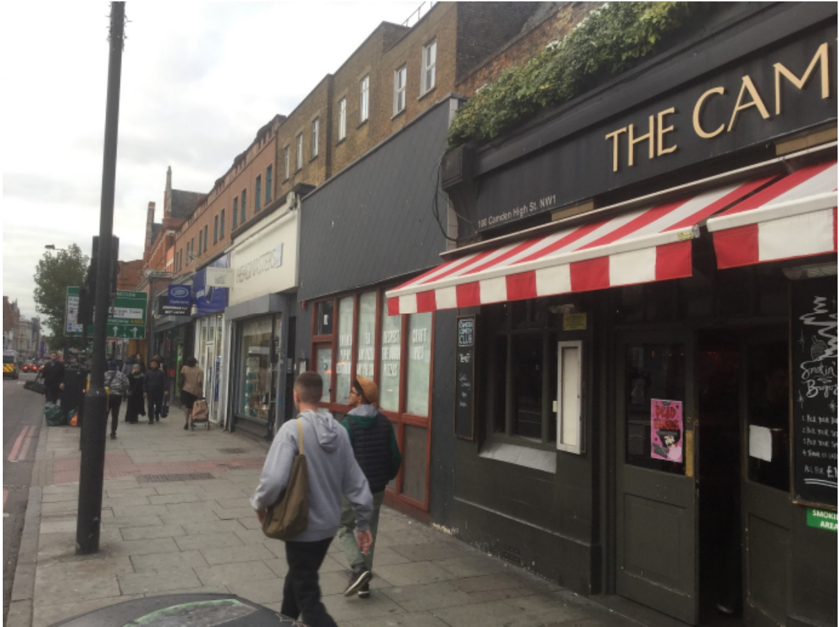
4. (Above) close up view of shopfront looking North.
