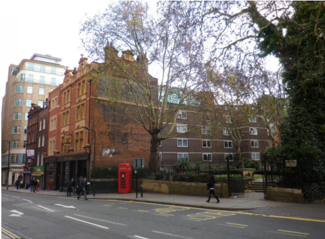
Photo 3 – View of rear elevation of building
