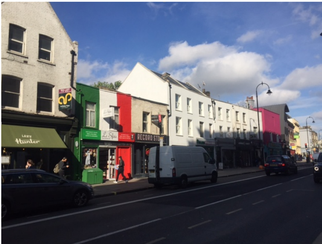
Photo 2 – Front elevations looking north
