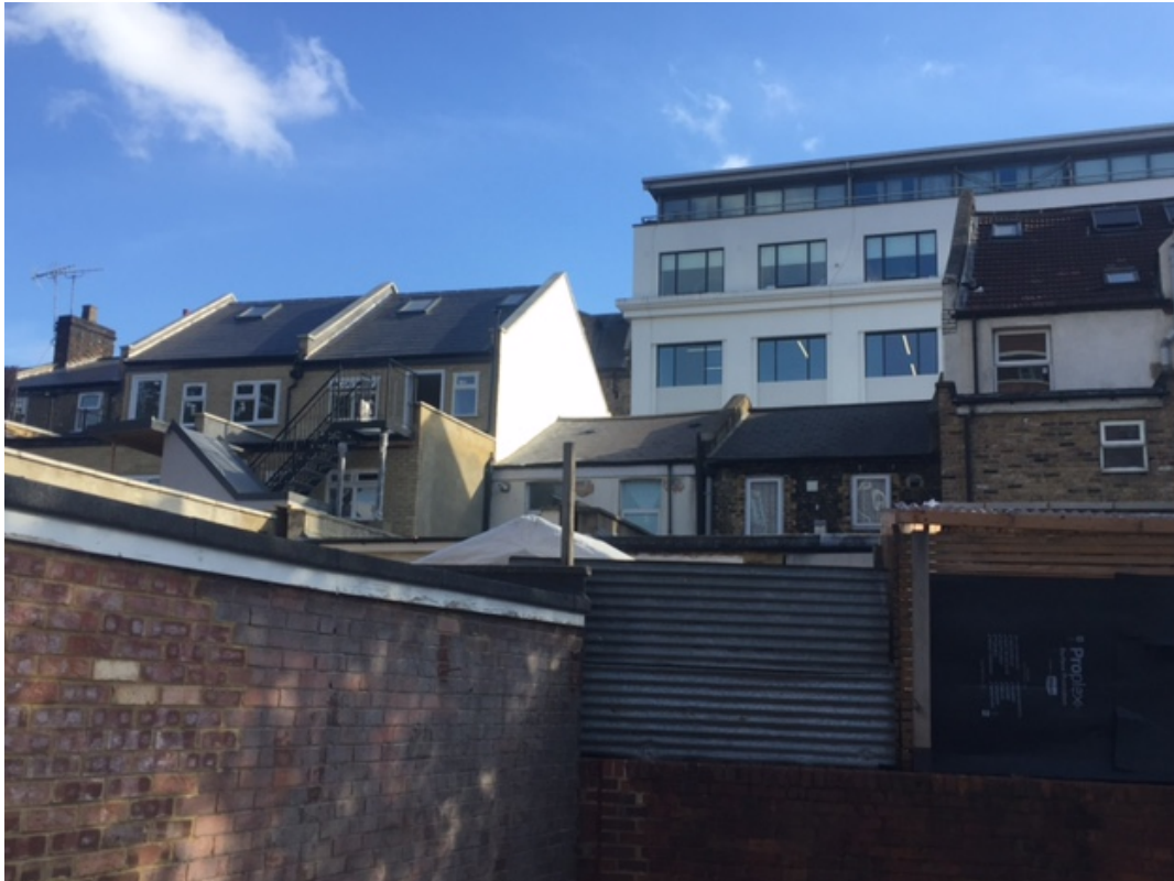
Photo 3 – Rear elevation of 117-125 as viewed from housing estate behind
