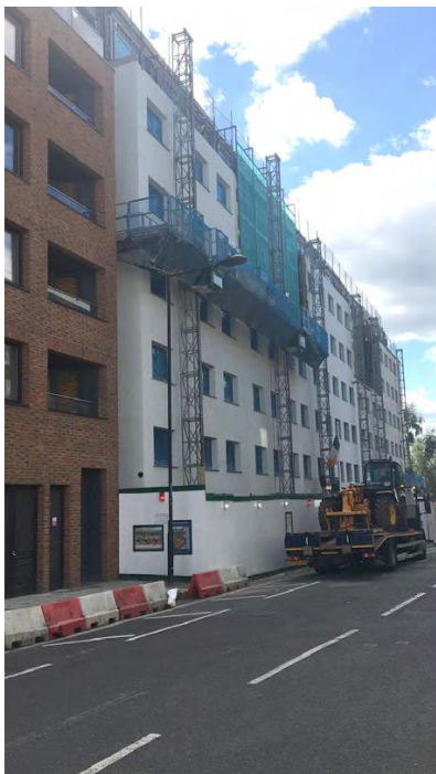
View north-east to south-west
