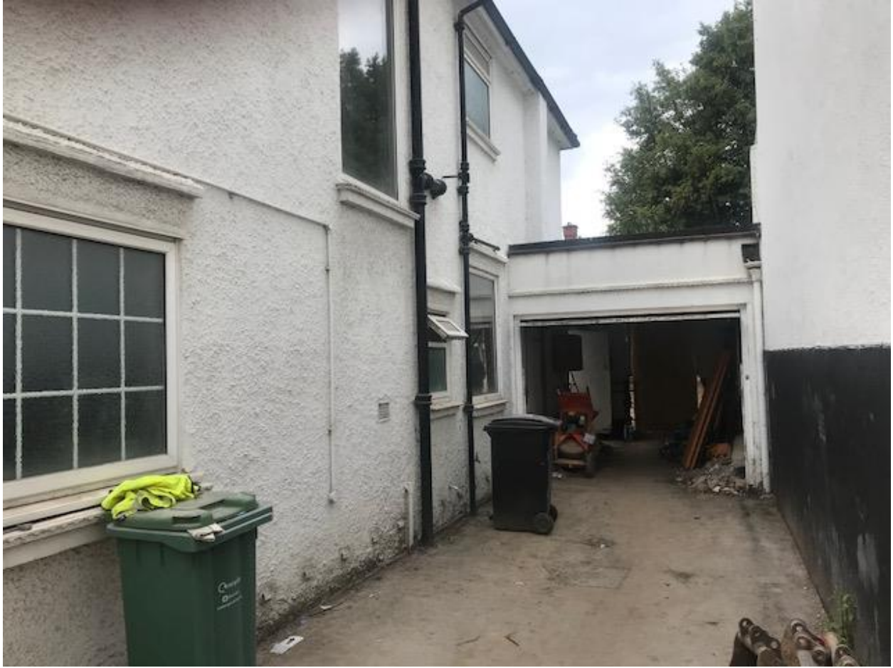
6. Existing side garage
