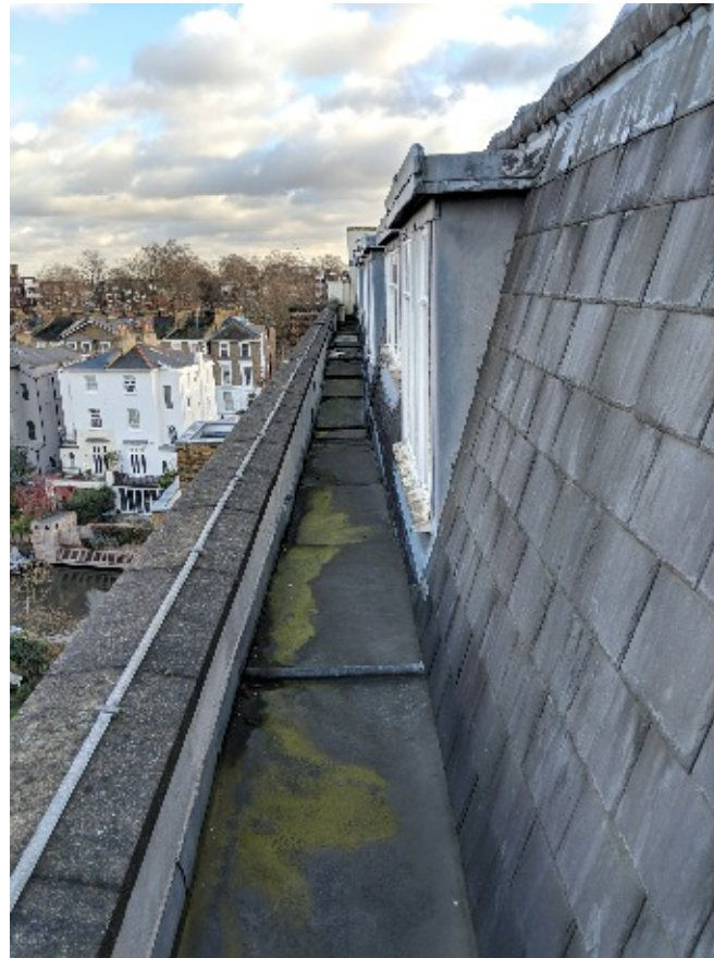
Image 07 Dormer windows on fourth floor
