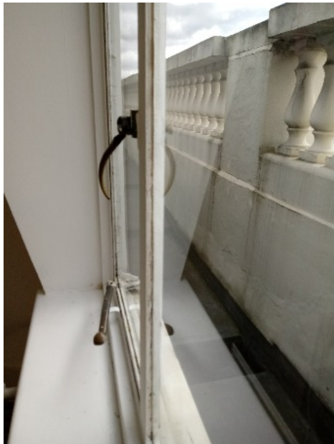
Image 10 Dormer windows on fourth floor - detail
