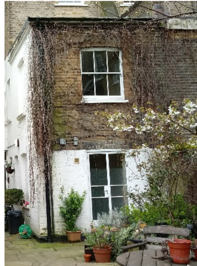
Image 08 Door to garden - Lower ground floor (external)
