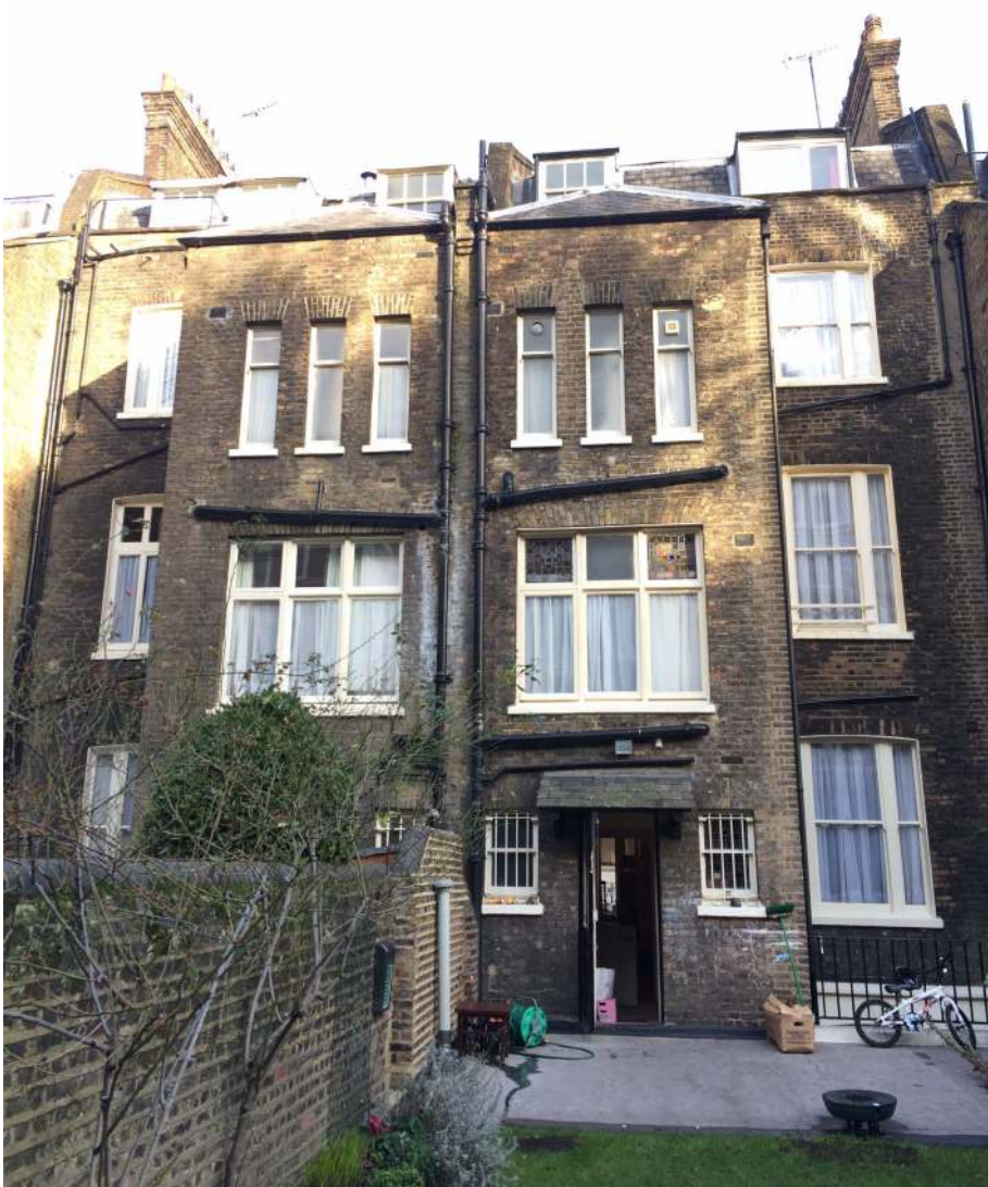
Figure 4: View of the rear elevation of nos. 65 (right) and 67 (left) Gower Street. Note the abutting closet wings / outriggers to each property which marks the centre of the terrace and where the existing shared bathrooms / WC facilities are located within no. 65.
