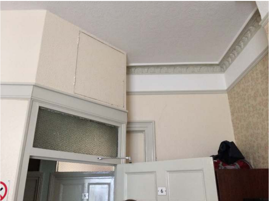
Figure 22: The former rear reception room at first floor level showing the harmful impact of the lobby partitions on the moulded plasterwork cornice and double door architrave which formerly opened into the front reception room.
