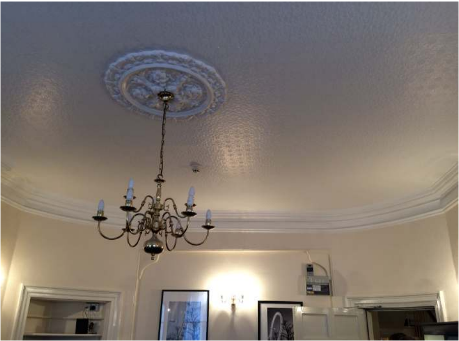
Figure 21: Former front reception room showing the curved walls to the inner corners. On the left this provides a void through which waste water could be routed from the proposed en-suite bathrooms to the rooms above without the need for any intervention through the ceiling or potentially harmful under-drawing.
