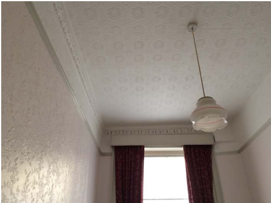
Figure 23 (above) and Figure 24 (below) - original part of the same front room the moulded plasterwork cornice has been partially removed within the northern compartment (above) this being the ornamental soffit shown below around the chimney breast. The removal of partitions would necessitate the restoration of the plasterwork soffit to ensure the legibility of the original space is suitably revealed and reinforced.
