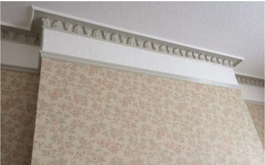
Figure 26: Plasterwork cornice to the rear first floor reception room with acanthus leaf and frond motifs.
