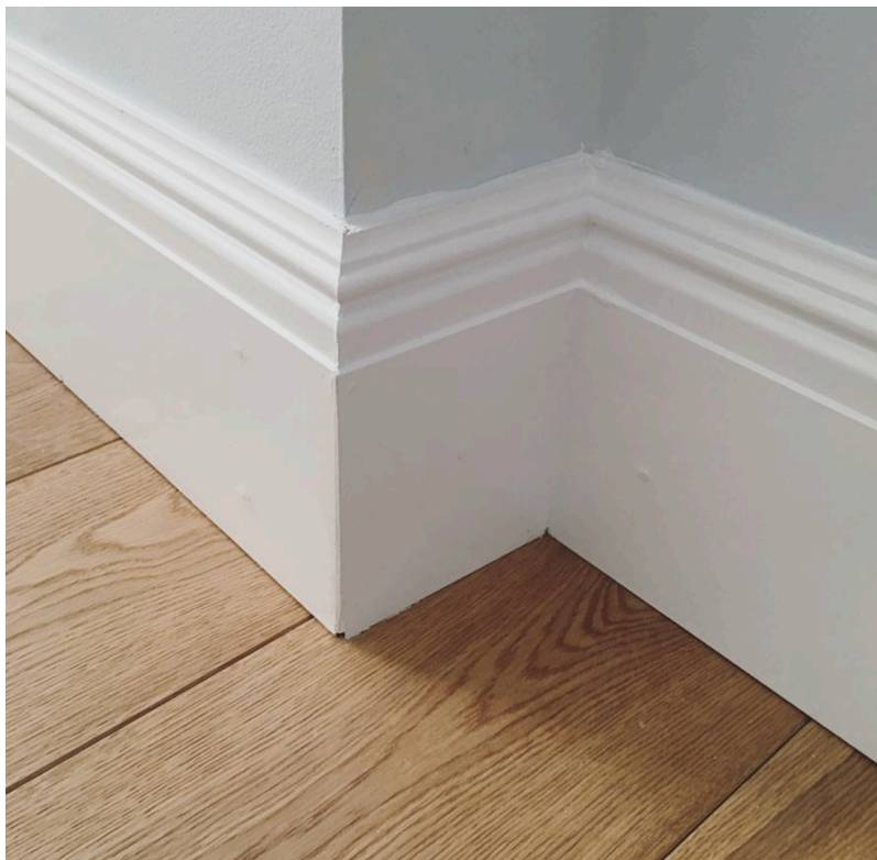
Photo.3 Proposed Skirting boards where necessary, are to match the existing exactly.
