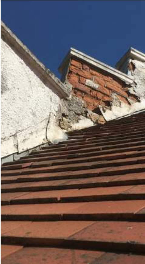
Roof parapets in poor conditions
