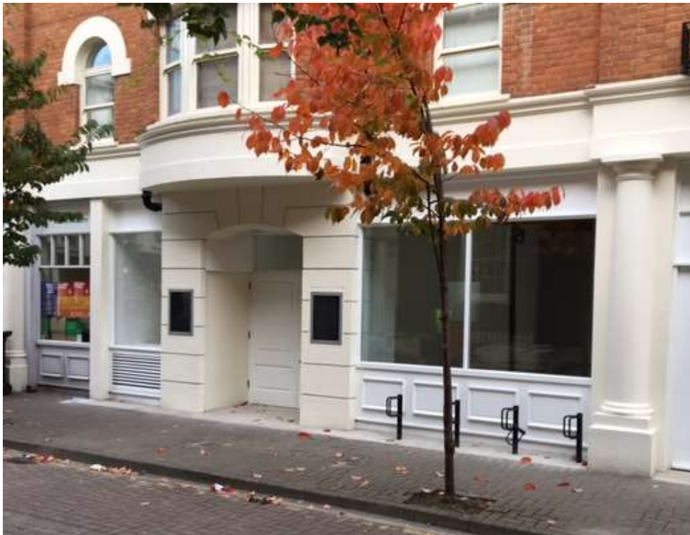
Existing Streatham Street frontage and entrance door to fitness studio
