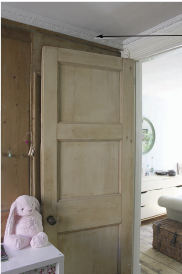
Upper ground floor, rear room
