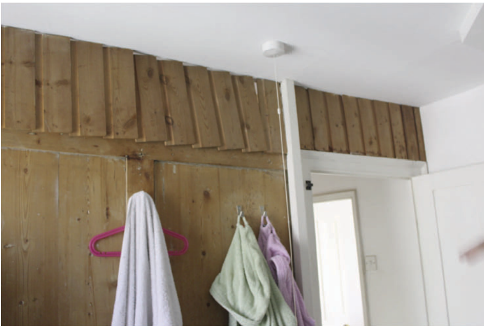
2nd floor rear bathroom
