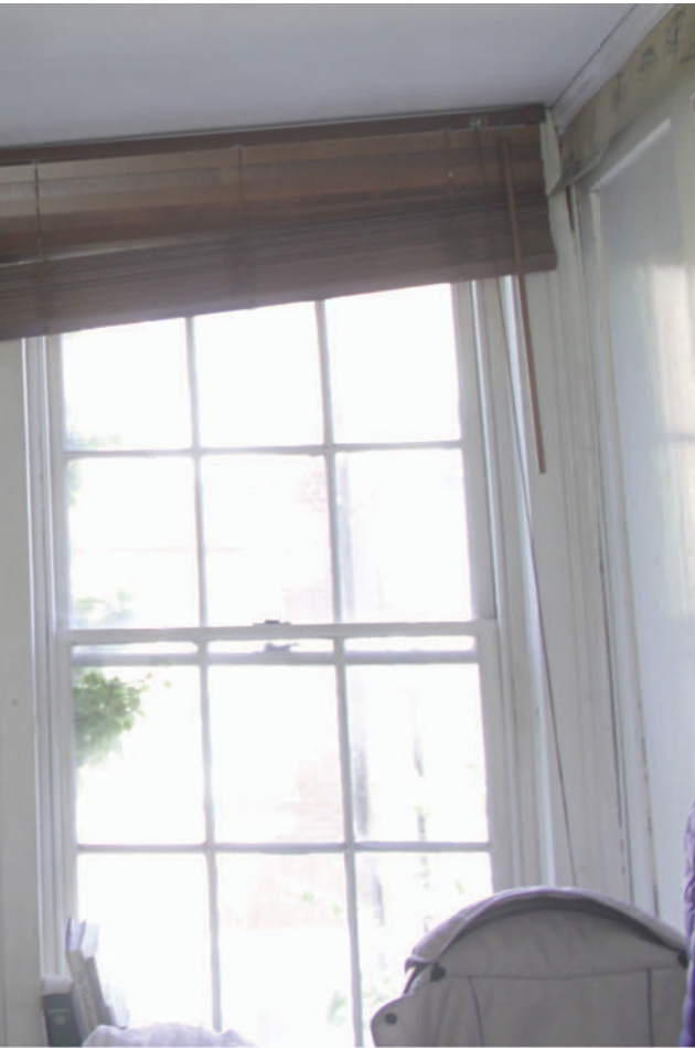
Window to first floor rear room
