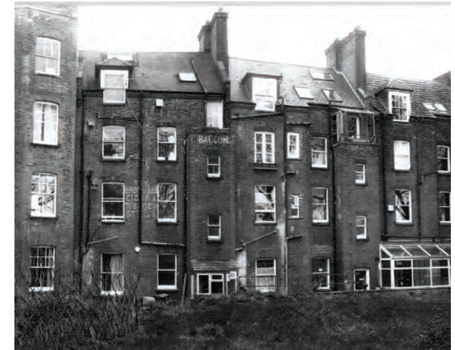
Rear elevations of existing buildings on Highgate West Hill, as taken from application 2006/2688/P
