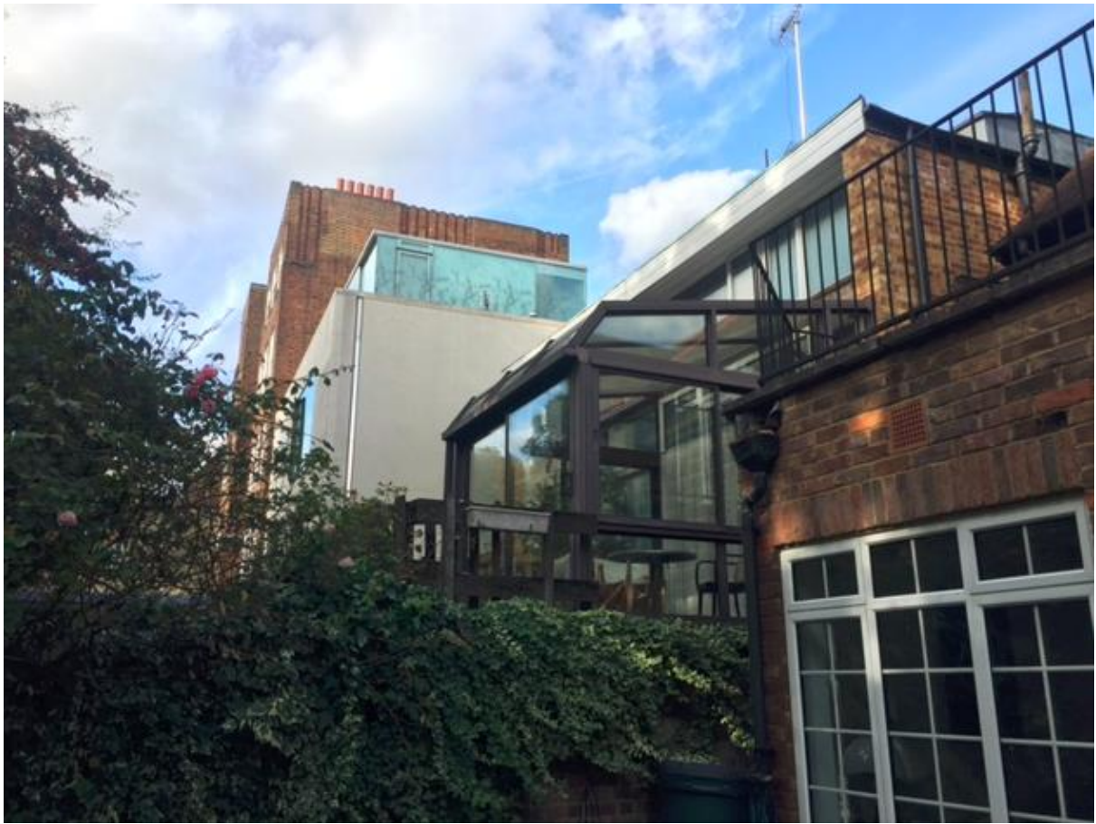
View 5 – Looking west towards neighbouring property 28b Glenilla Road
