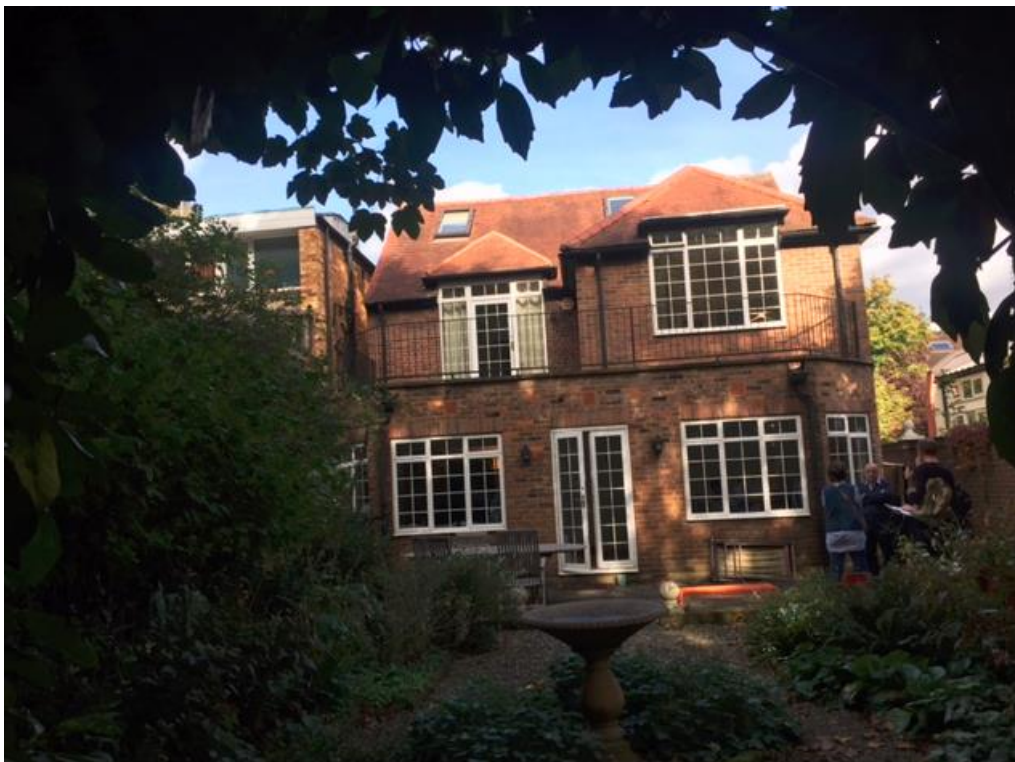
Photo 4 – View of rear elevation
