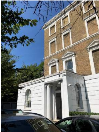
Side elevation, exposed to the south west
