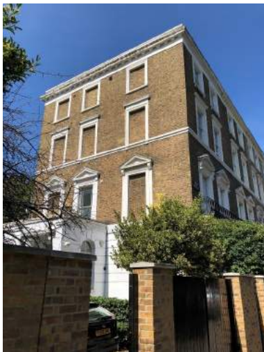
A view from the west, side elevation exposed
