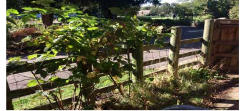
Proposed boundary treatment to match existing: timber post and rail with dog mesh, continuous hedge planting, metal railing self-closing gates
