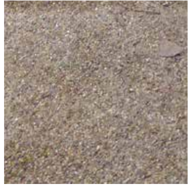
Tarmac surface with amber aggregate to match main park path
