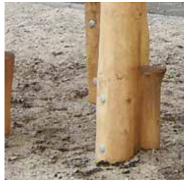
Robinia posts with stainless steel bolts and shoes
