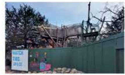
Timber hoarding fencing 2.5m high
