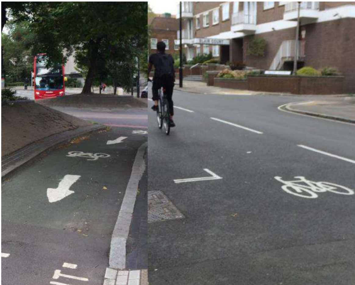
Photograph 3 Cycle Lane and Markings
