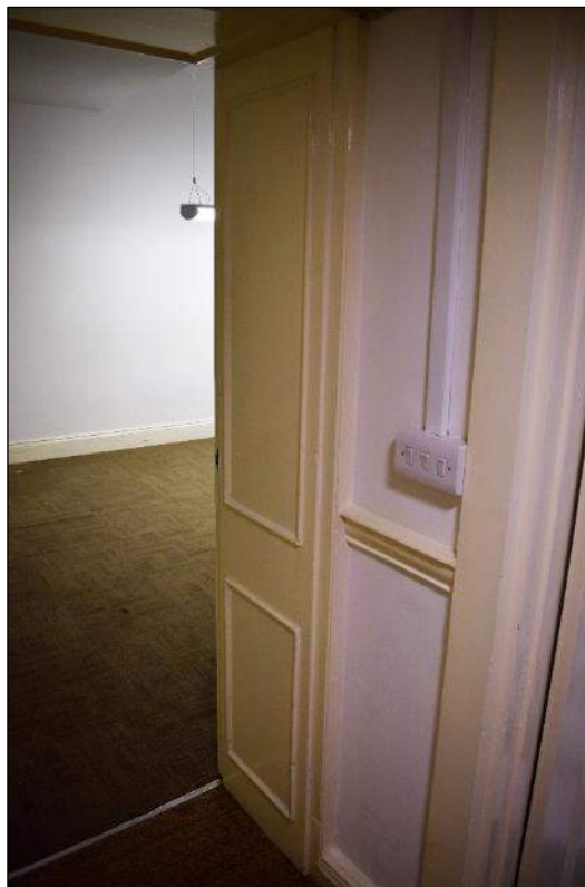
Photo 6: Wood panelling, dado rail and original skirting
