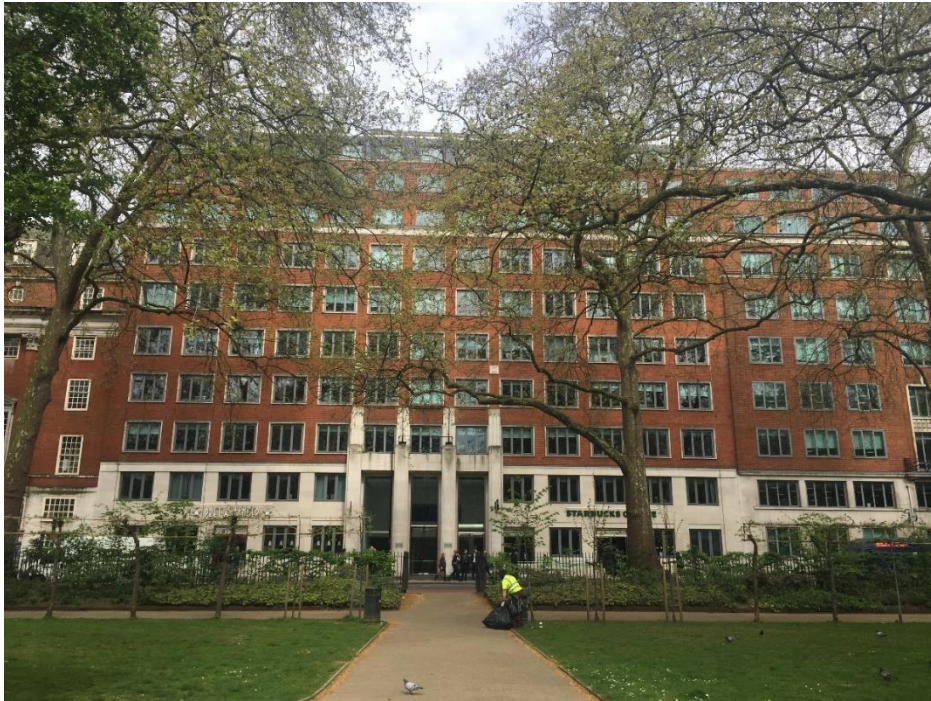
Figure 2: Lynton House, front elevation as seen from Tavistock Square
