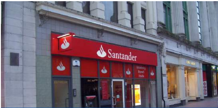
Basement damp proofing at Santander Bank, Marylebone
