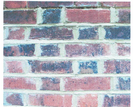
▲ Very bad pointing in grey cement mortar. The mortar is smeared over the face of the bricks and the work is untidy.
