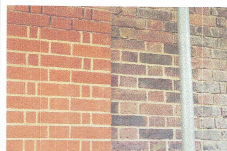
▲ The brickwork to this house had been very poorly repointed. The illustration shows that with painstaking and highly skilled craftsmanship this can be put right. This is repointing of the very highest standard. It is necessarily expensive but greatly enhances the appearance of the house and will have a positive effect on its value.
