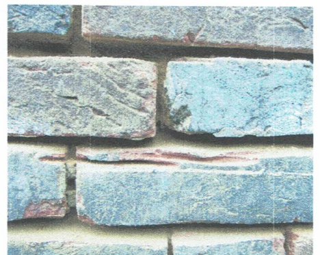
▲ Bad cutting-out with a mechanical grinder. The bricks have been badly damaged and the joints widened.
