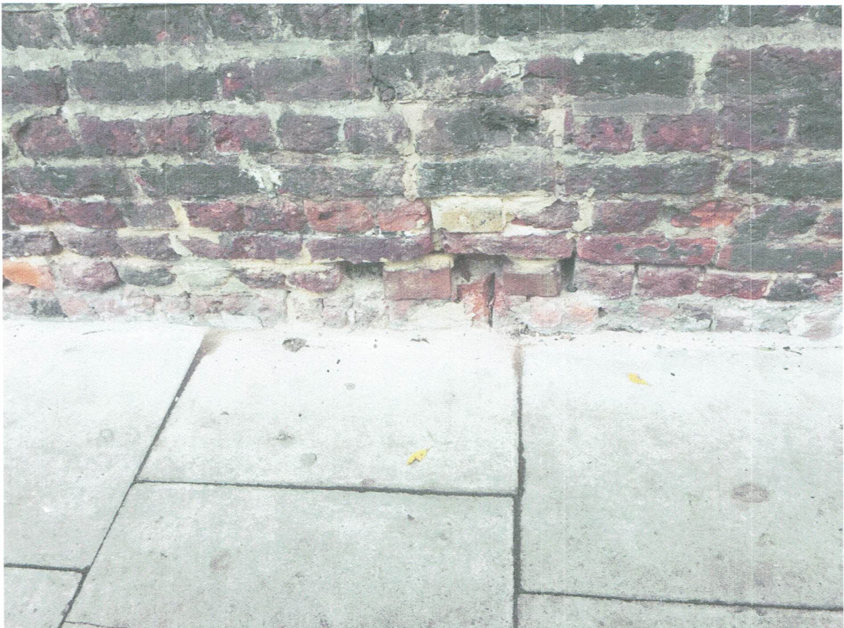
Typical damage caused by de-icing salts
