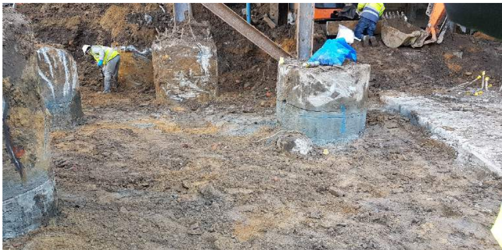
16/02/2018: Soils at formation level in contaminated area, prior to removal.
