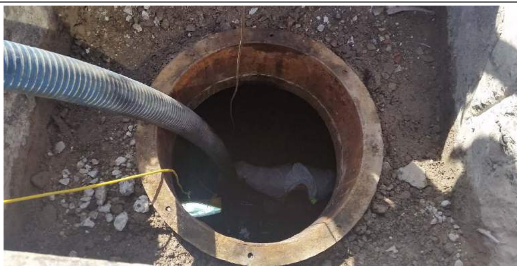
Man entry into tank for cleaning and suction of sludge.
