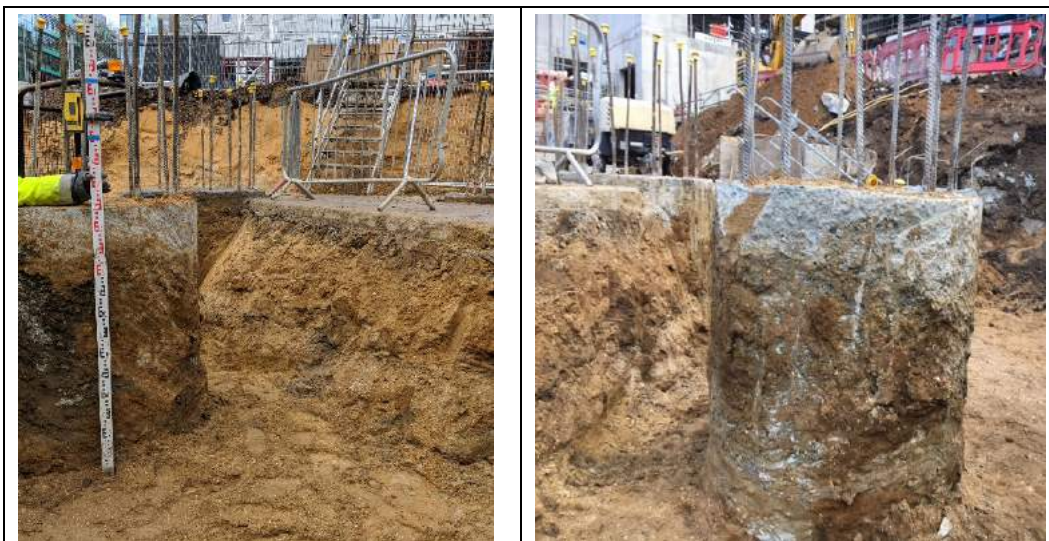
20/02/2018 (left) and 22/02/2018 (right): Remediation excavation to 1.2m below basement formation level. No obvious visual and olfactory indicators of hydrocarbon contamination noted in the base or sidewalls of the excavation..
