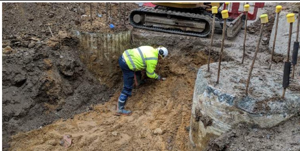
06/03/2018: Collection of the final verification sample from eastern side of the remediation excavation. The final sample was carried out following extension of the excavation following a failed sample.
