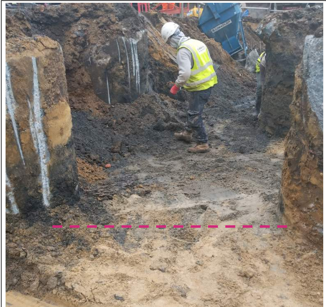
09/02/2018: Excavation works within contaminated area. Annotated line on shows boundary between “clean” and contaminated soils at the proposed basement formation level. Excavation and removal of the visually impacted soils was subsequently carried out.
