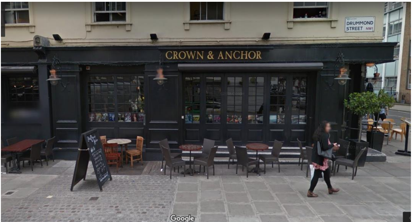
EXISTING FAÇADE SHOWING EXISTING BI-FOLDING DOORS AND FIXED WINDOW TO LEFT HAND SIDE (Above)
