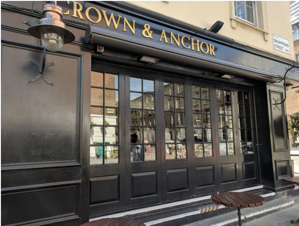
EXISTING BI-FOLDING OPENING DOORS (Above)
