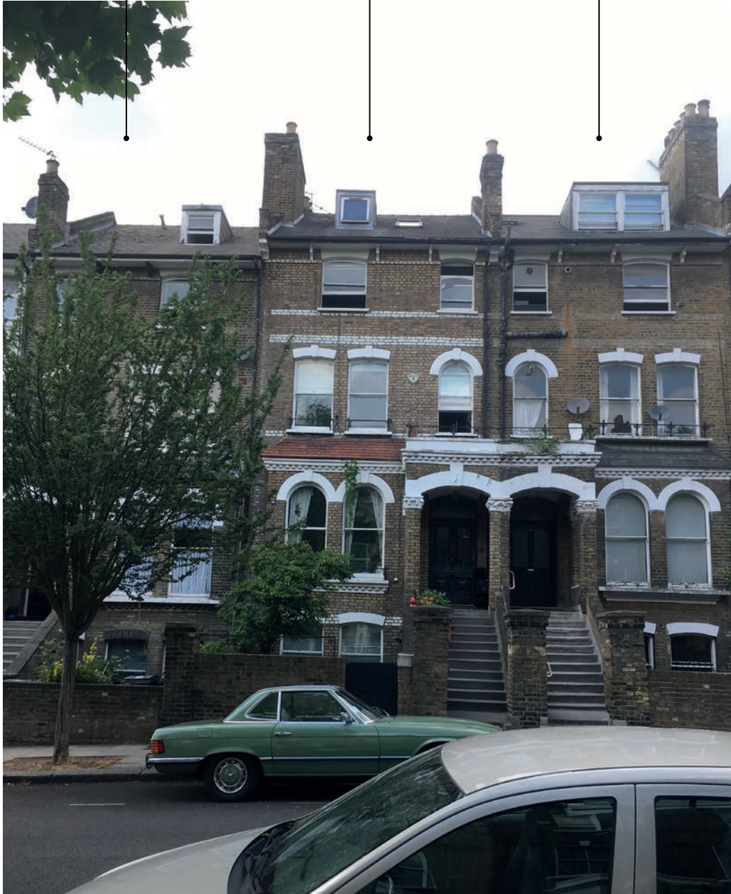
View of 81 St Augustine's Road street elevation.
