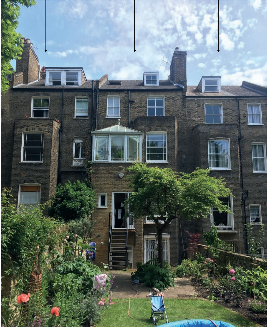
View of 81 St Augustine's Road rear elevation. Existing extension to be remodelled.
